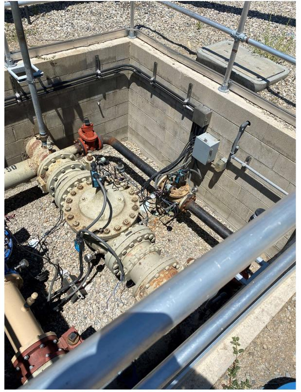
Figure 15 Cla-Valve Flow Control Valve at Agate Reservoir
