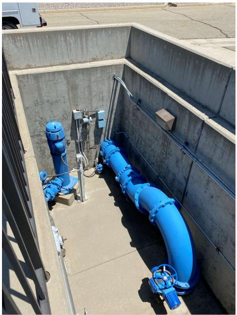
Figure 5 Hinckley WTP Flocculation and Sedimentation Basin Inlet
