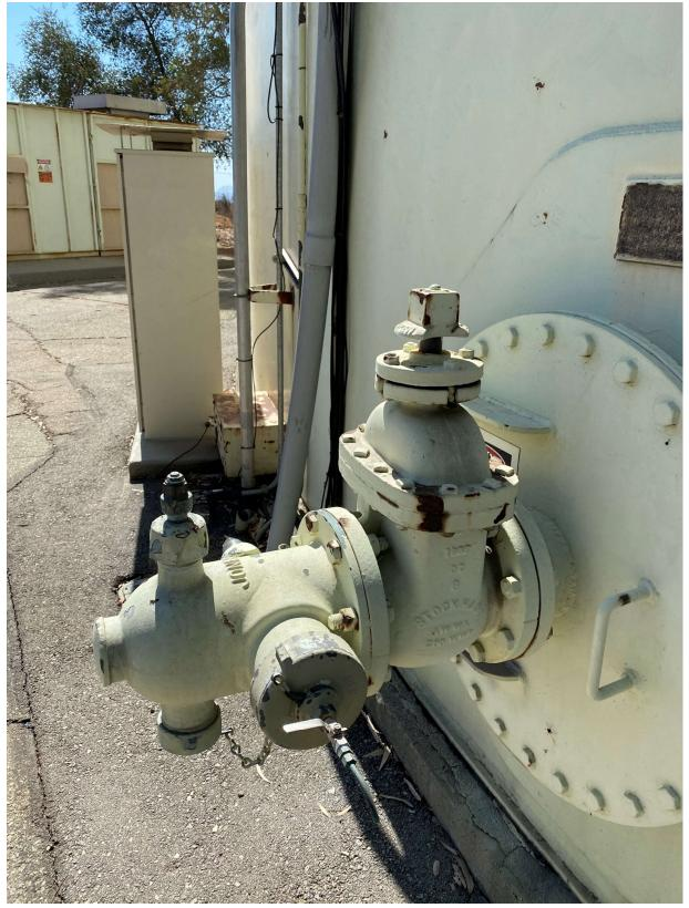
Figure 48 Access Manhole Valve is Corroded
