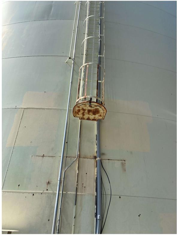
Figure 43 Steel Shell is Spot Corroded-Attached Ladders are Rusted Beyond Repair
