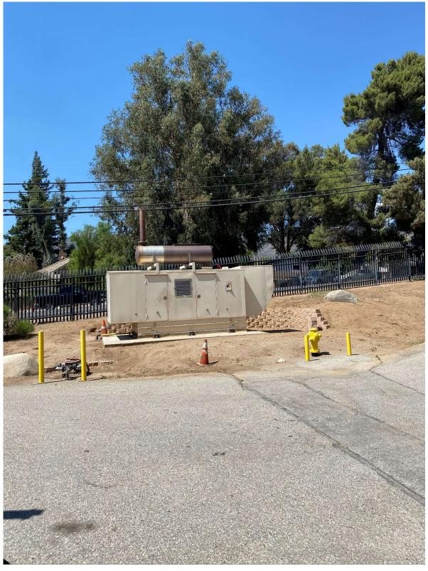
Figure 33 Standby Diesel Generator Set
