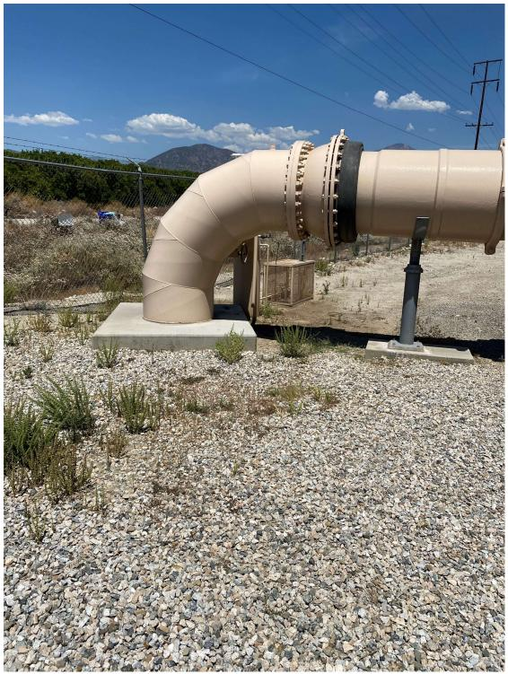
Figure 16 Agate Reservoir Seismic Expansion Unit Supported Off the Concrete Slab
