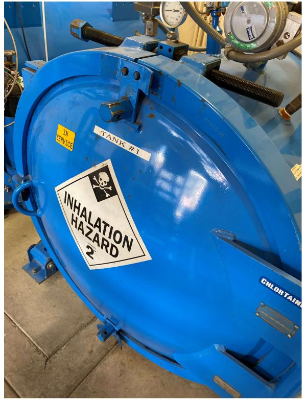
Figure 30 Safety Enclosure of the Chlorinators
