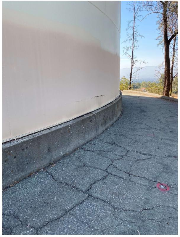
Figure 46 Reservoir Base (surrounding asphalt is cracking and evidence of deterioration)
