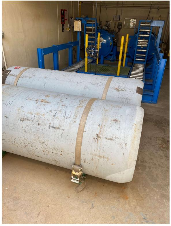
Figure 31 Chlorine Cylinders Stored Onsite
