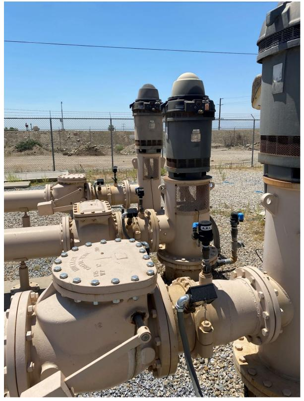
Figure 23 Booster PS Discharge Valves and Pressure Gauges
