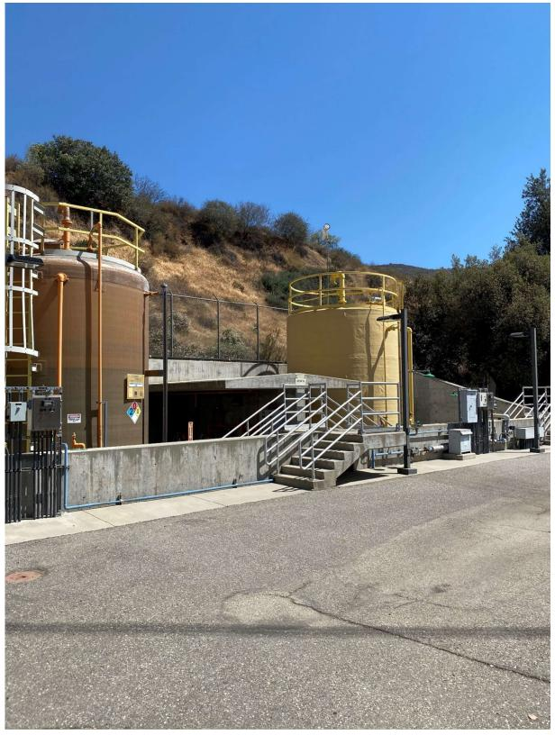
Figure 35 Chemical Storage Area with Concrete Containment-In Good Working Condition
