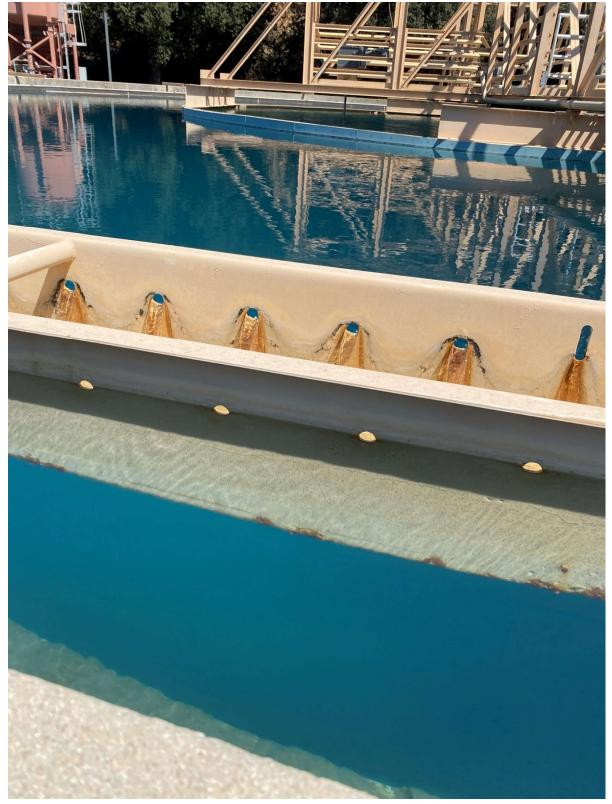
Figure 37 Eimco Settler (Signs of Aging and Corrosion of Mechanical Equipment)
