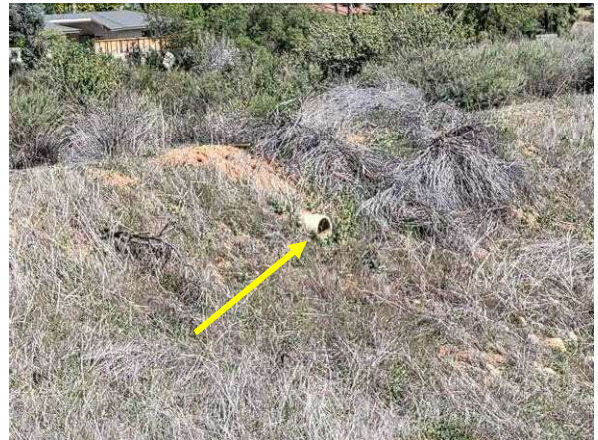
Photo #4 View of storm water drainage pipe (concrete), located on the central portion of the site.
