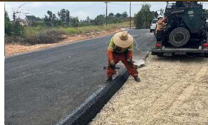
Installing asphalt dike on Fairmont Dr.
