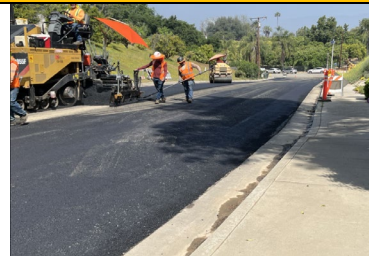
Contractor paved Marvin Avenue
