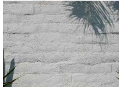
SACK FINISH WALL EXAMPLE
