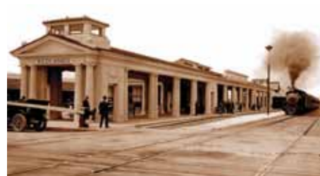
Early Redlands developed with centers of civic and economic activity located near transit opportunities.
