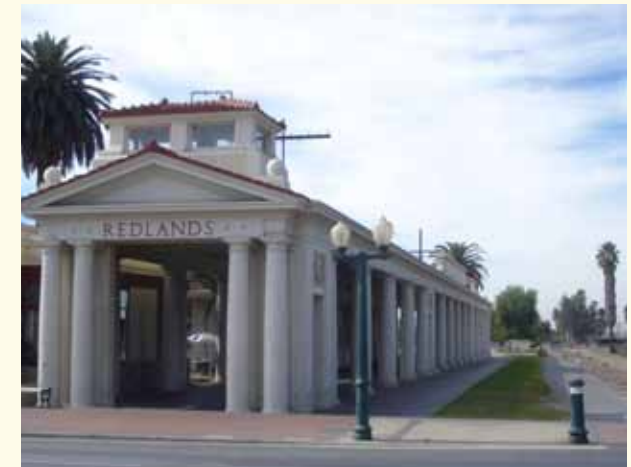
The Redlands Rail Depot once welcomed rail passengers to the city. Though the Depot today is not part of the Redlands Passenger Rail project, it remains an icon of Redlands.
