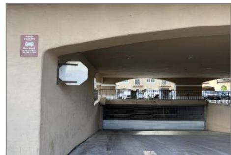
Entrance to Centennial Plaza Garage
