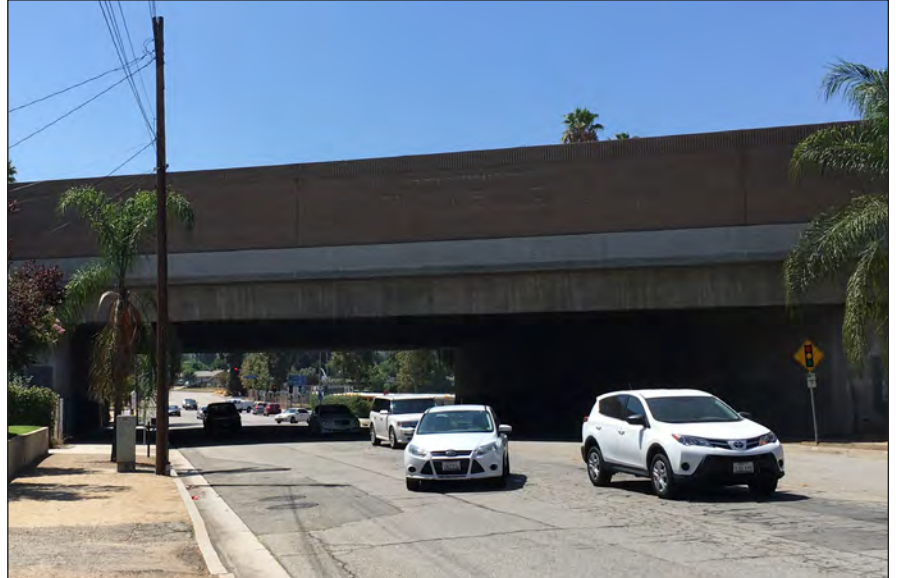
The inadequately lighted University Street freeway underpass.
