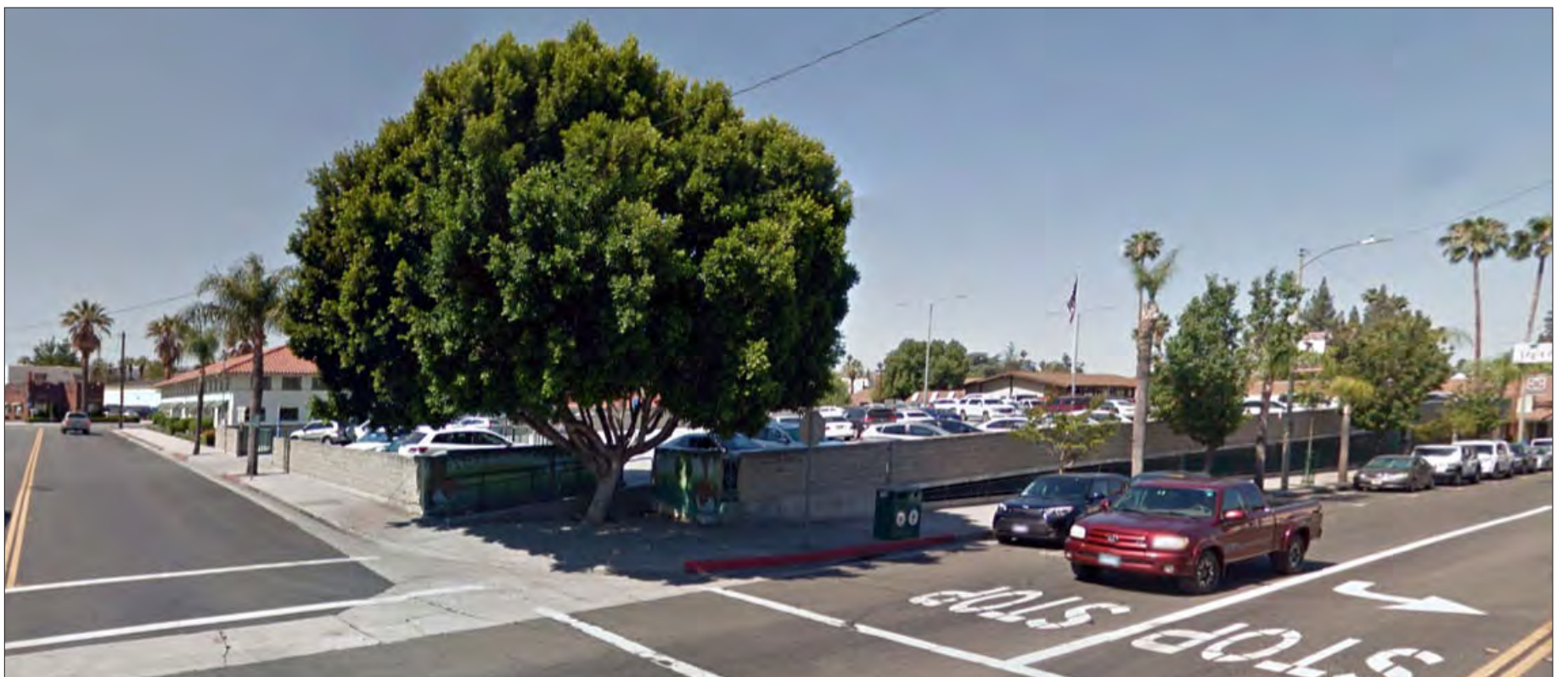
View of City-owned Citrus Avenue parking garage.
