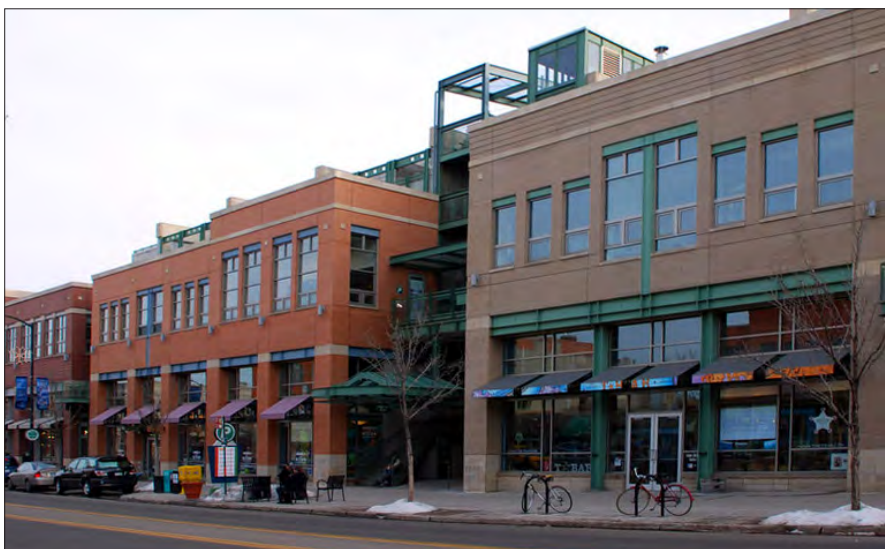
Access to this lined parking garage is directly from the sidewalk.
