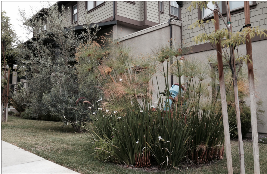
A back flow preventer that is located immediately adjacent to the building and is screened from the view of the sidewalk and street by shrubs.
