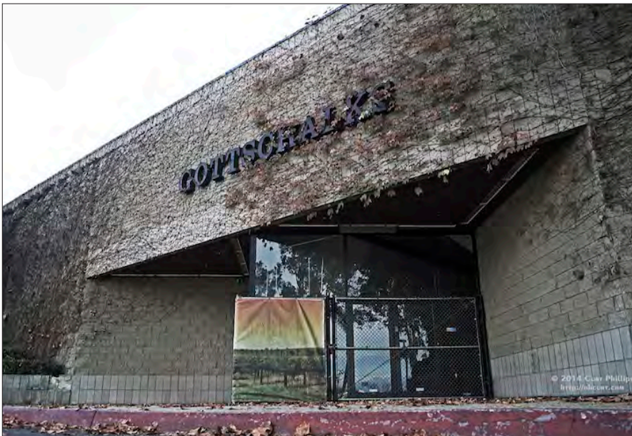
The entrance to the Gottschalks entrance, boarded up since 2009.
