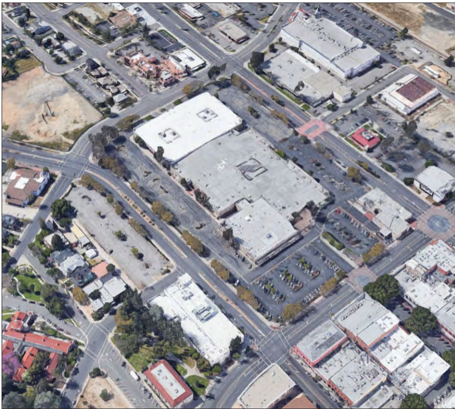
Bird's-eye view of the existing Redlands Mall site.
