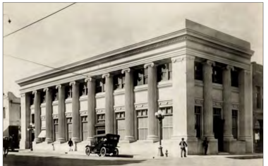
The First National Bank Building, originally located on the southwest corner of State Street and Orange Street, was demolished in 1975.
