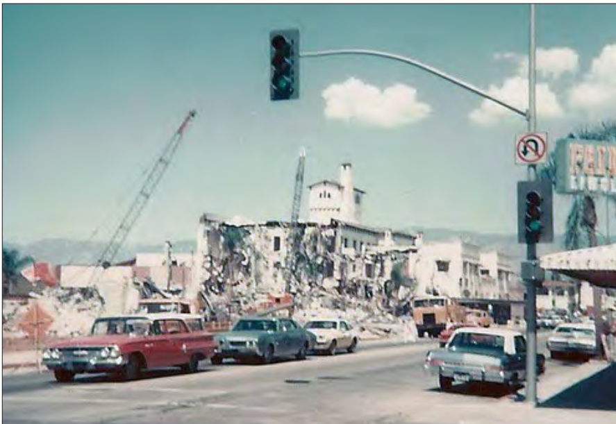
The demolition of the First National Bank Building.
