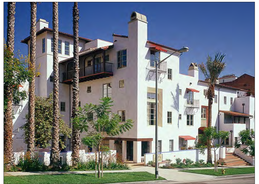
A multi-family building with varied floor heights.
