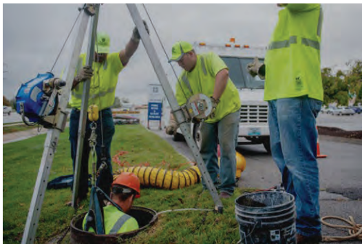
Photo 1.1. Confined Space Entry
