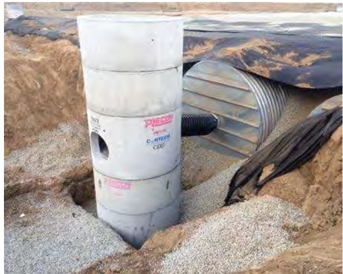
The CDS® provides direct access to cleaning, using a combination of swirl concentration and indirect screening.
