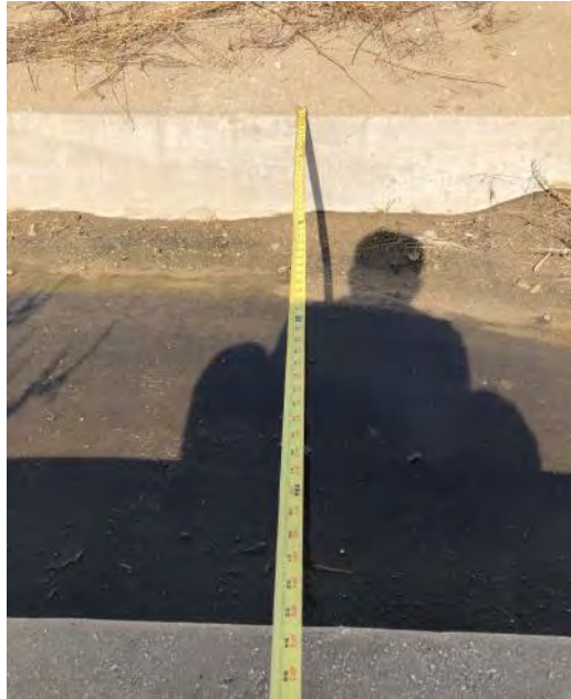
Photograph No. 7: U-shaped concrete structure trending east-west along center line of future extension of Pennsylvania Avenue is about 4.5 feet wide and 12 inches in height
