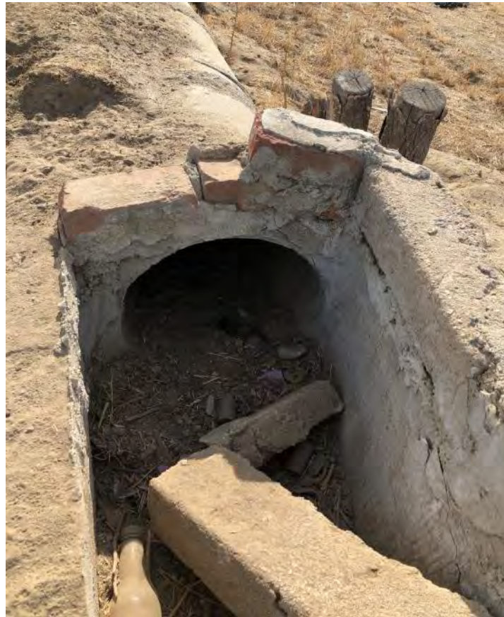
Photograph No. 9: Viewing south along west side of site showing concrete drainage structure (U-shaped structure in foreground and circular concrete pipe in background)
