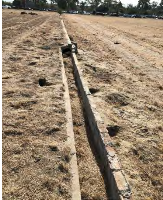
Photograph No. 9: Viewing south along west side of site showing concrete drainage structure (U-shaped structure in foreground and circular concrete pipe in background)
