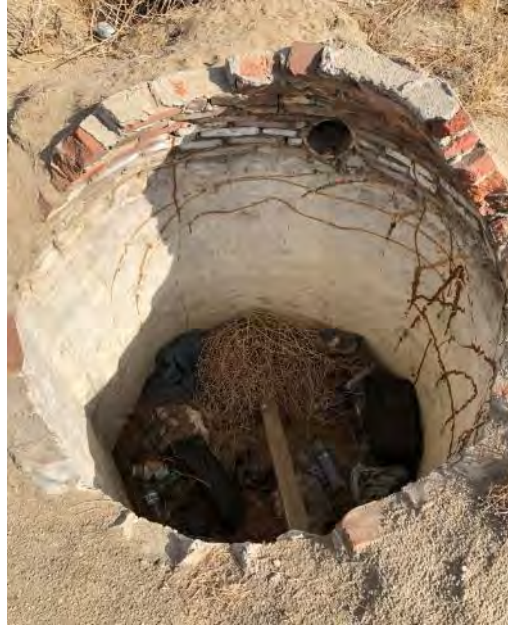
Photograph No. 13: Open cylindrical excavation (shaft) made of brick, concrete and filled with debris in the southwest portion of the site
