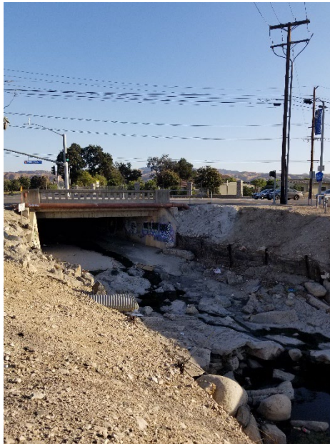
Photograph 2. Looking Southeast at Mission Zanja Channel and existing bridge over California Street. Improvements and widening of the existing bridge will occur here.
