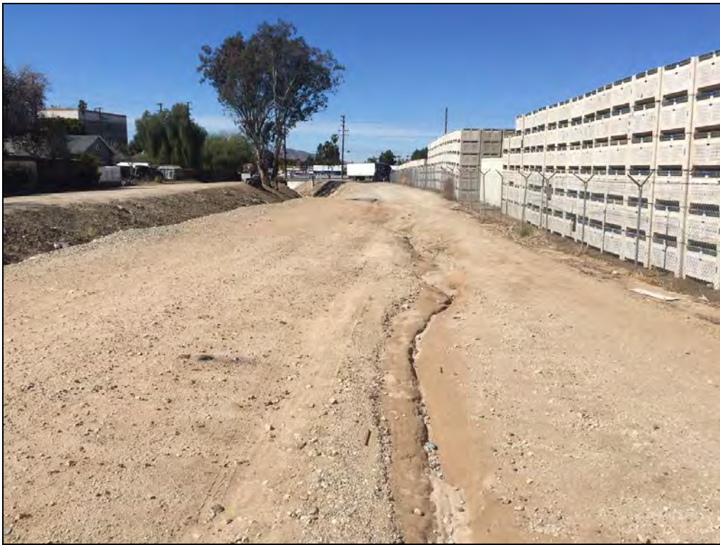
Photo 8: Erosional feature located on the proposed Zanja Trail; facing west.
