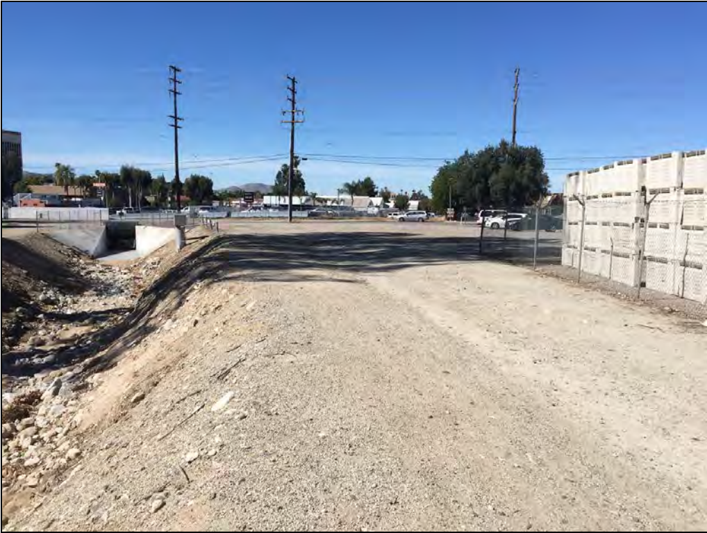
Photo 4: Proposed location of Zanja Trail north of Zanja channel (disturbed area); facing west.
