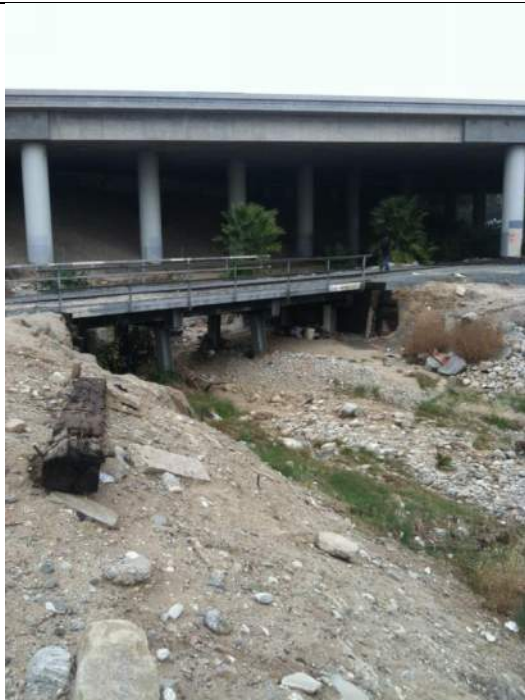
Zanja Creek – Railroad crossing
