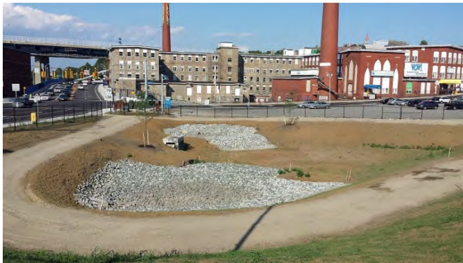
Infiltration basin in an urban area. The basin has two gravel areas for infiltration. The remainder of the basin bottom and its slopes are planted with sod.
