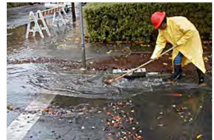
Clogged Storm Drain
