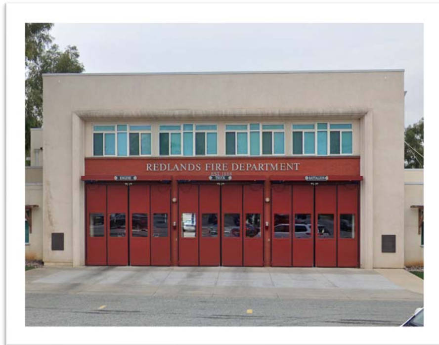
Station 261 Brand New Bay Doors
