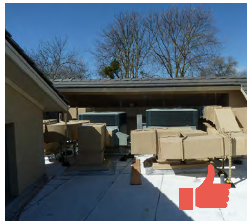
This mechanical equipment is located below the parapet of the building so that it is not visible from the public right-of-way.
