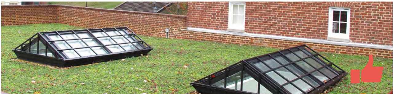
An example of a green roof with appropriately scaled vegetation that does not extend above the parapet.
