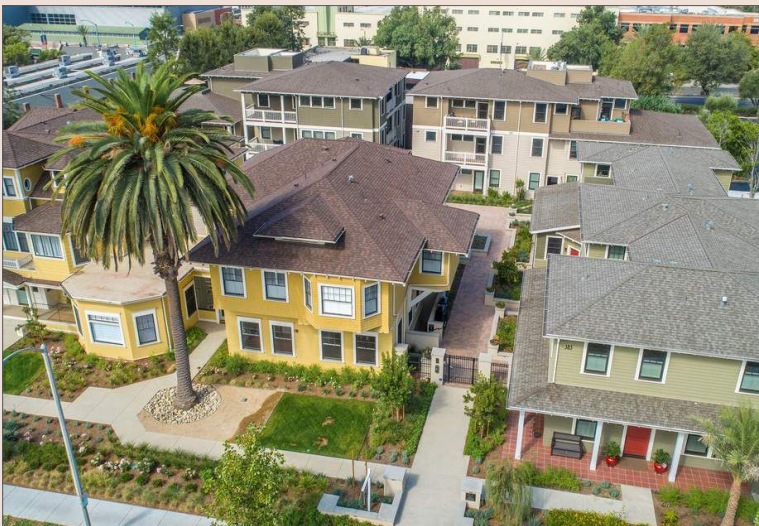
Individual buildings designed with different massing, frontage elements, and wall and window colors. Taller buildings are at rear of site.
