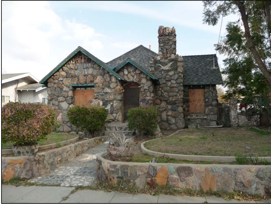
Example of a Stone Building, 2017.
