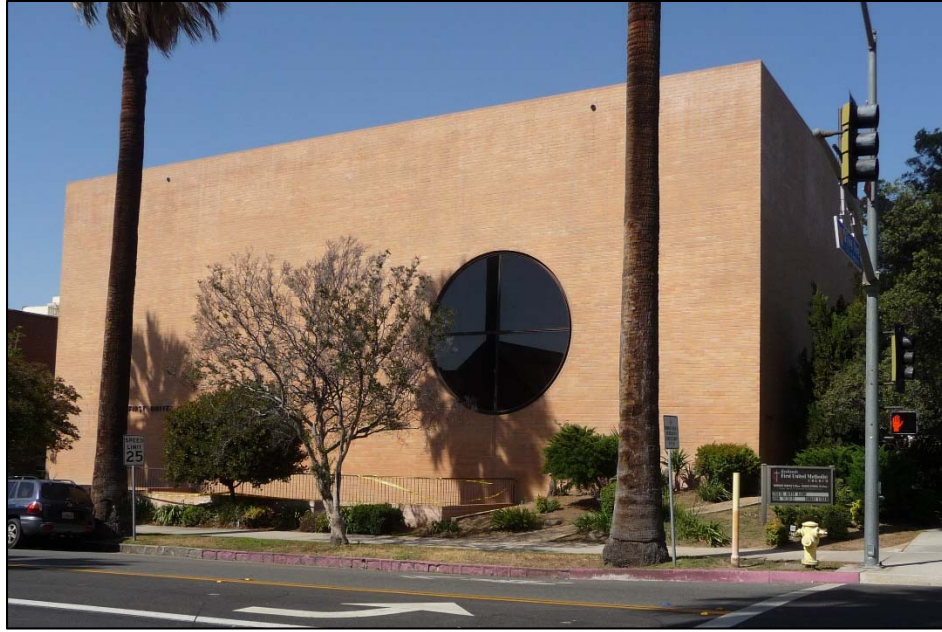
First United Methodist Church (1970), 1 E. Olive Avenue, 2017.
