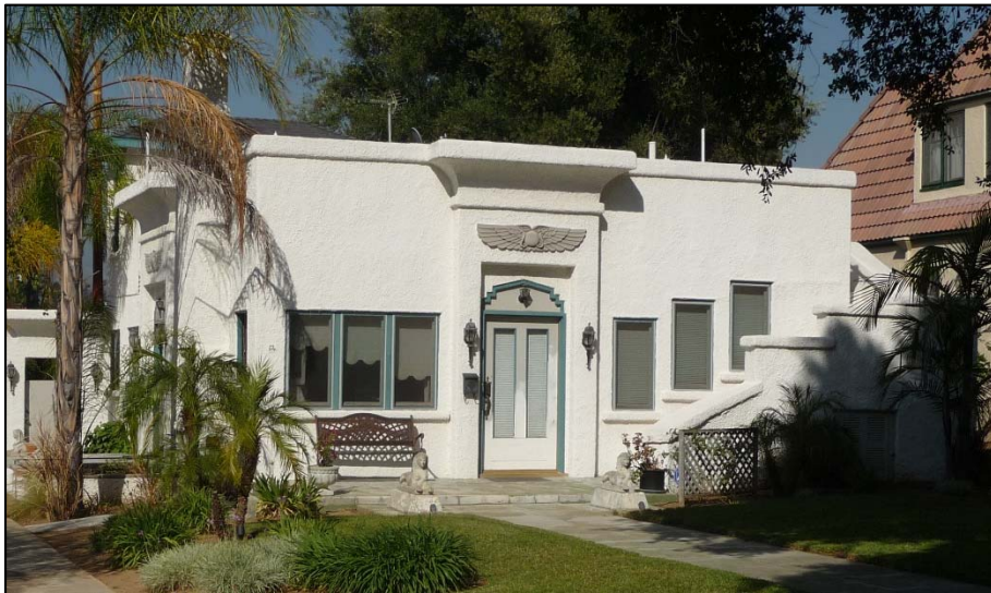
Example of the Exotic Revival style (Egyptian Revival), 2017.
