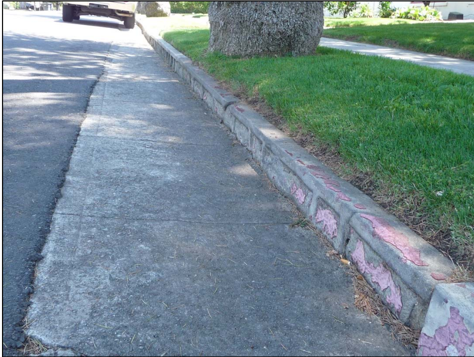
Stone curbing, Grant Street, 2017.
