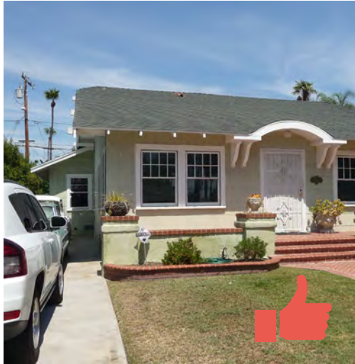
An example of an appropriate addition to a historic building. The addition is located on the side façade, set back from the front of the building; it is smaller in footprint and subordinate to the main building, and its roofline has a similar pitch as the historic roof pitch.
