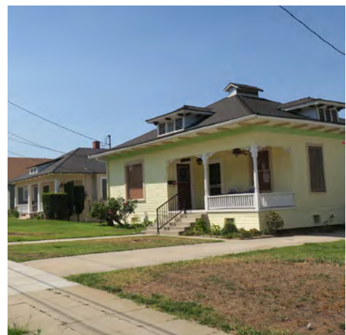
A row of Victorian style cottages.
