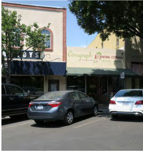
Most commercial buildings in Redlands have flat roofs.
