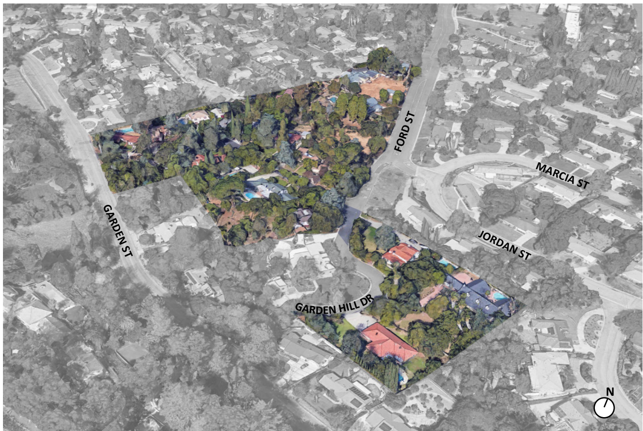
Aerial looking up Ford Street toward the northwest.
