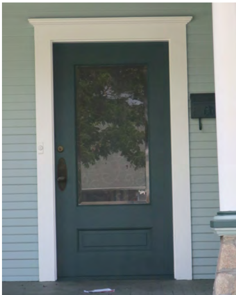
Single wood doors with paneling and glazing are common features of pre-war houses in Redlands.
