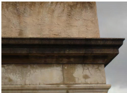
Repair and maintain historic architectural features, such as this cornice, to prolong its life.
