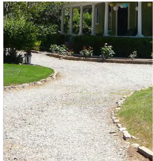
Porous driveways help with water runoff.
