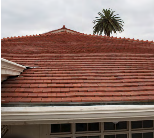
Clay tile (terra cotta) roofing on the Santa Fe Depot.
