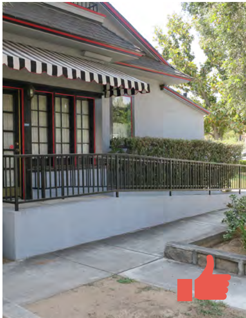
The accessibility ramp at the side of this building is painted and retains a simple design that is compatible with the historic building.
