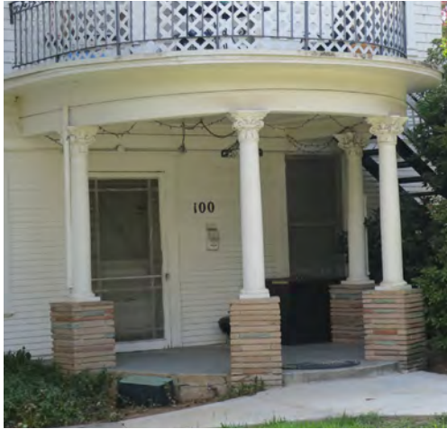
Restore non-historic porch components, such as these piers supporting original porch columns, to their original condition.
