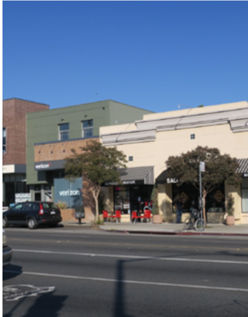
New commercial designs should be distinctive but compatible with the historic block context.
