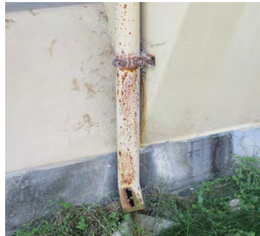
Corroded downspout.
