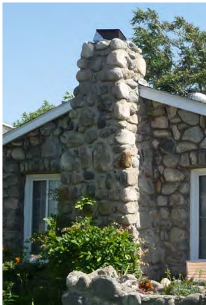
Exterior stone chimney.
