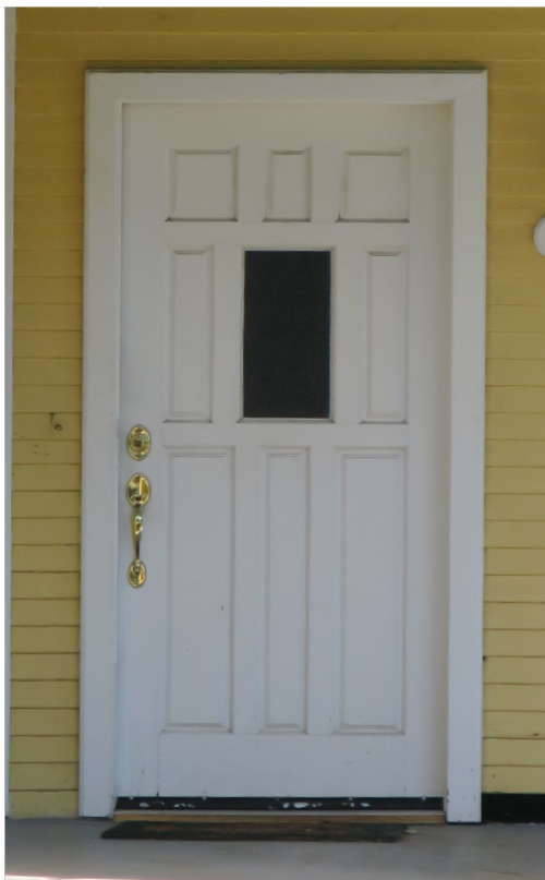
Maintenance, such as repainting and adding new glazing putty, will prolong the life of a historic door.
