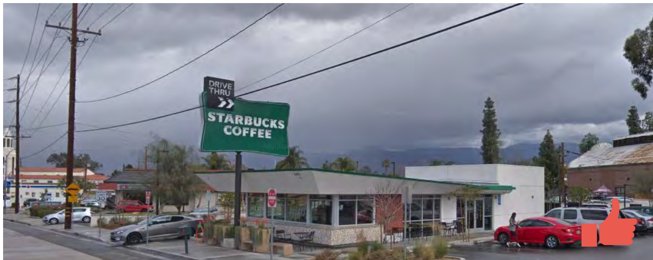
A simple one-story rear addition is compatible with the scale and design of this historic drive-thru restaurant. (Image, Google, 2018)
