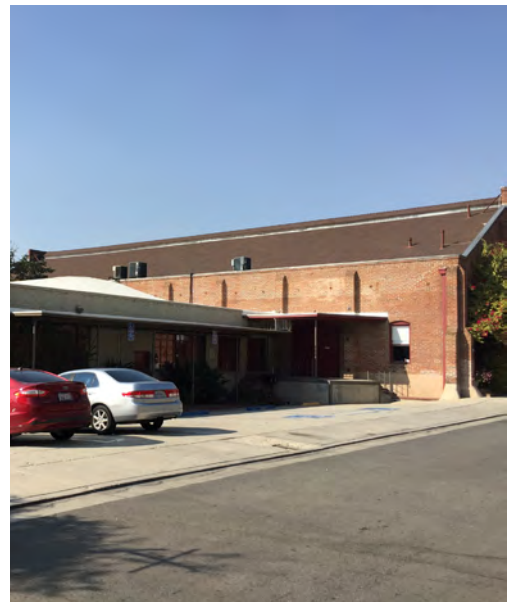
An example of side parking at an industrial building.
