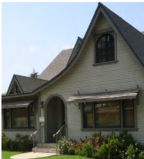
Awnings are a historically appropriate solution to keeping a building cool.
