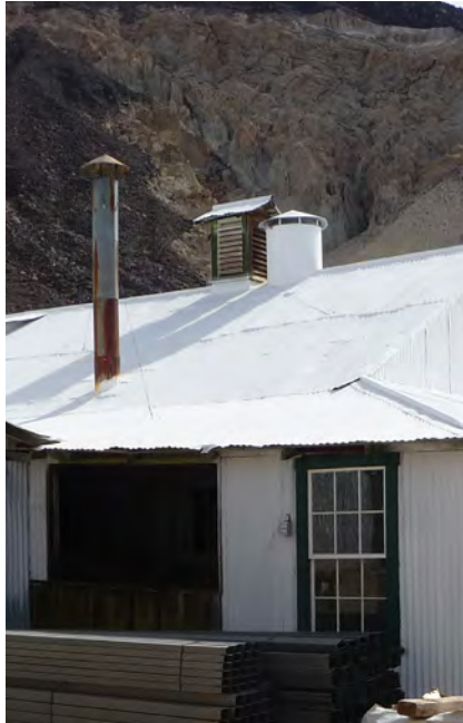
Roof with multiple penetrations and flues.
