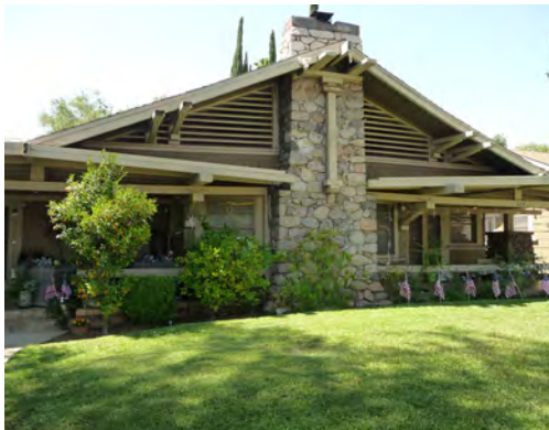
Wood roof details on a Craftsman duplex.
