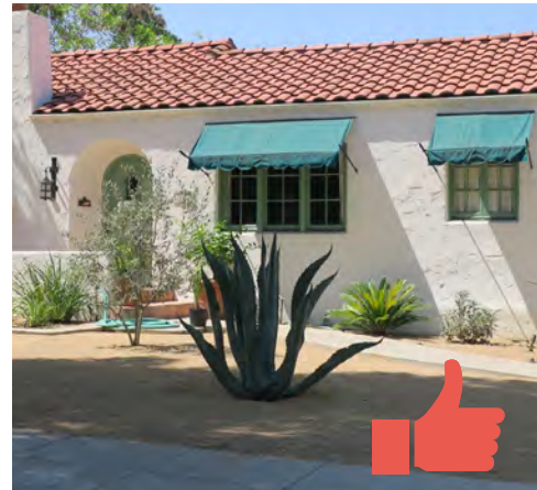
These new valance and picket awnings are historically appropriate for a Spanish Colonial Revival style house.
