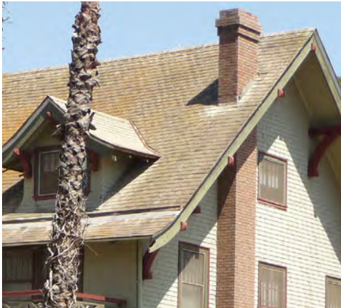
Inspect seismically vulnerable historic components, such as chimneys, to ensure they are structurally sound.
