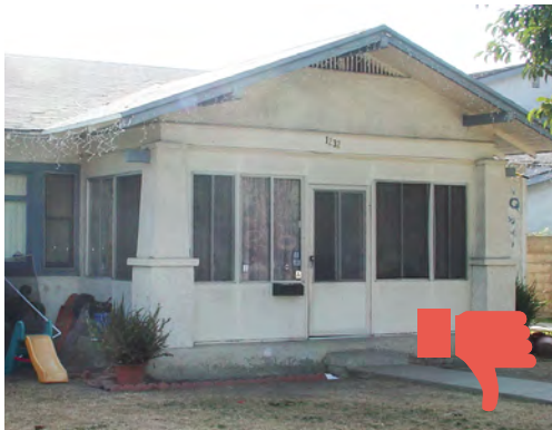
Avoid enclosing a historic porch at the primary entrance to the building.
