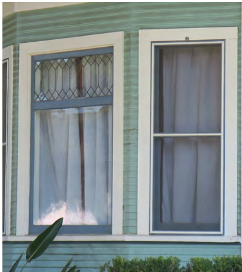
Seek less invasive weatherizing solutions first, such as installing interior curtains or shades.
