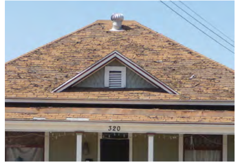
Replace a historic roof only when it is deteriorated beyond repair.
