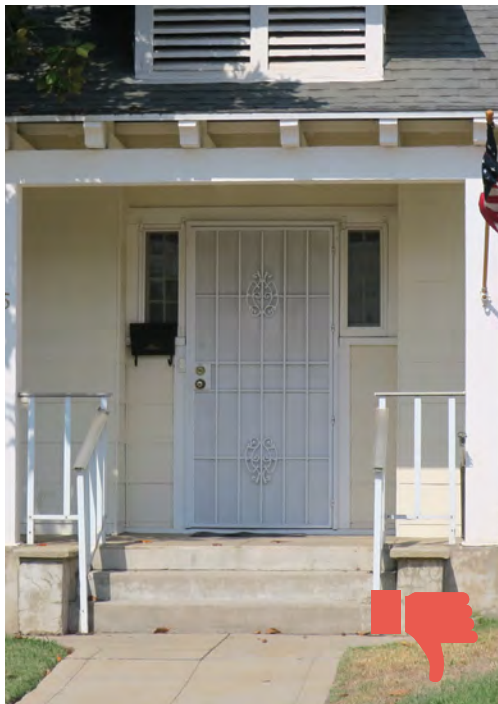
Avoid installing a metal security door that obscures the original historic door from view.
