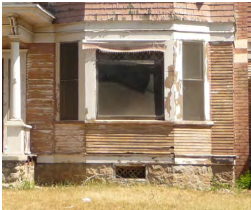
Repair historic windows when the physical condition warrants additional work.
