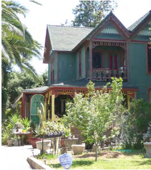
Decorative gingerbread details and multi-colored shingles are defining features of Queen Anne and Stick architecture that should be preserved.
