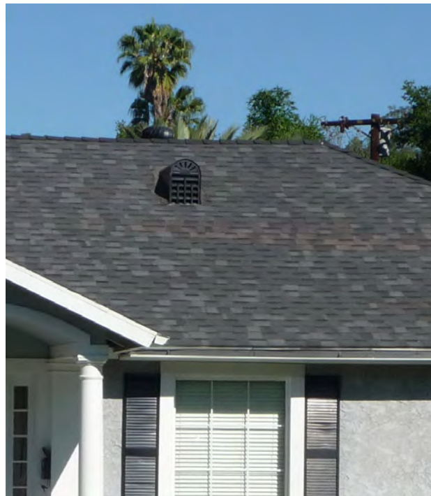
Composition shingle roofing.
