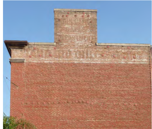
Restore a missing historic sign, such as this painted sign, based on historic documentation.
