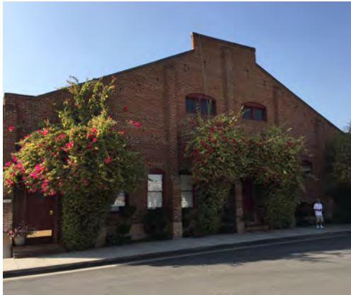
Brick pilasters provide some articulation to this industrial building.
