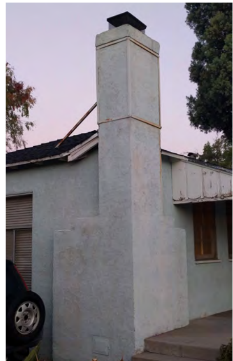
Brace or reinforce chimneys.
