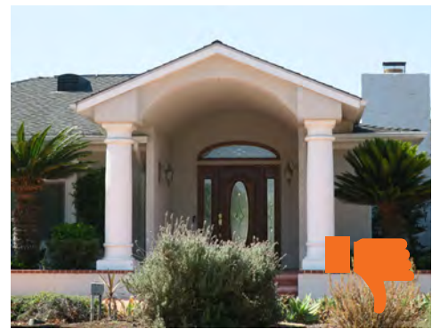
Avoid adding new features that are not appropriate to the architectural style of a building, such as classical columns on a Ranch style house.
