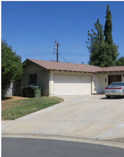
An example of an attached garage, a common characteristic of the city's postwar residences.
