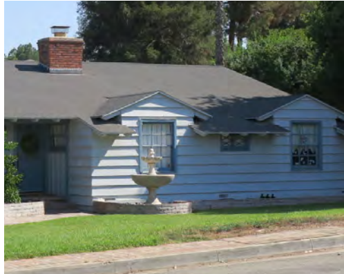
An example of the types of windows and doors that are appropriate for Redlands' postwar neighborhoods.
