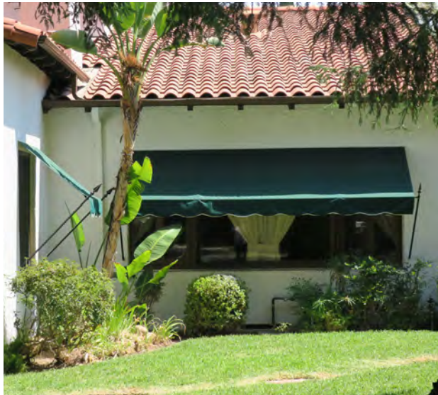
Decorative metal awning supports.
