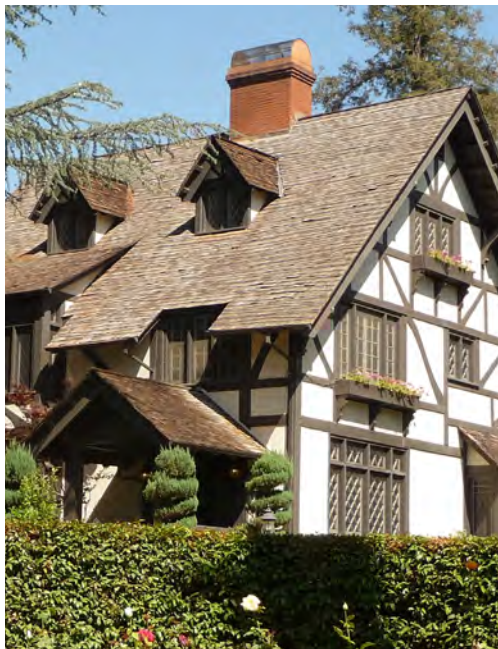
Routine maintenance is the key to preserving a wood shingle roof.
