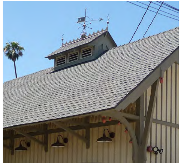
Decorative metal finials and weathervane at roof ridge..
