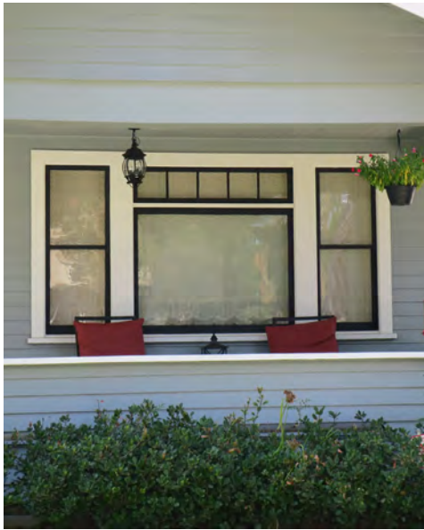
Vertically oriented, double-hung wood windows are typical of houses in the city's pre-war neighborhoods.
