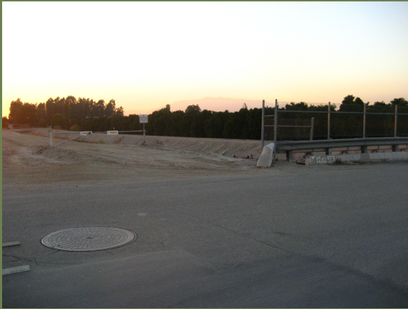
Zanja Creek at Nevada St. facing west
