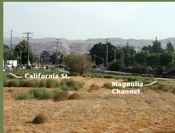
Magnolia Channel approaching intersection of California St. and Redlands Blvd. facing south.
