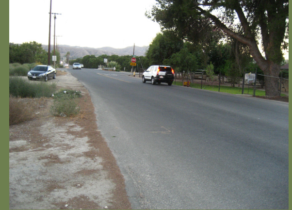
Zanja Creek at New Jersey St. facing south
