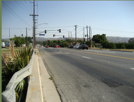
Zanja Creek at Alabama St. bridge - toward Citrus Ave.
