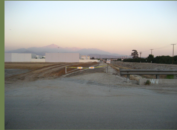
Zanja Creek at Nevada St. facing east
