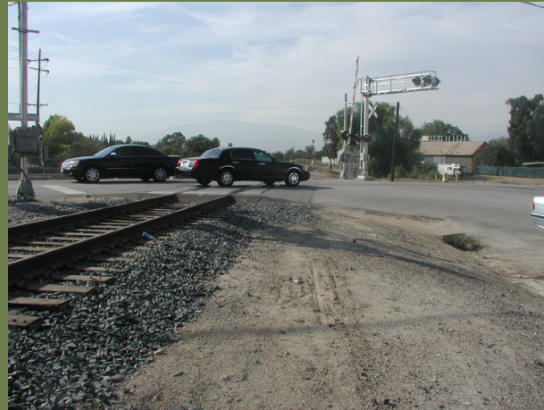
Railroad tracks at Mountain View Ave. facing west
