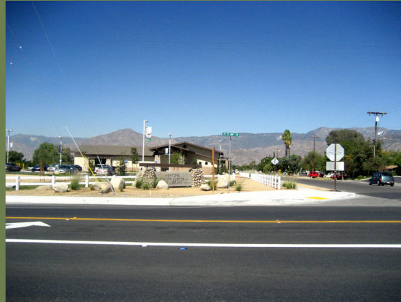
Mentone Sr. Center/Library at the intersection of Opal Ave. and Wabash Ave. facing north toward the proposed Santa Ana River Trail
