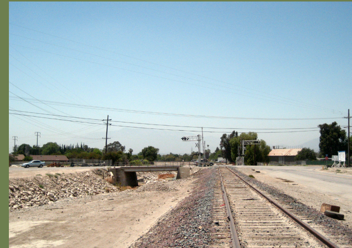
Mountain Ave. automobile bridge viewed from upstream.
