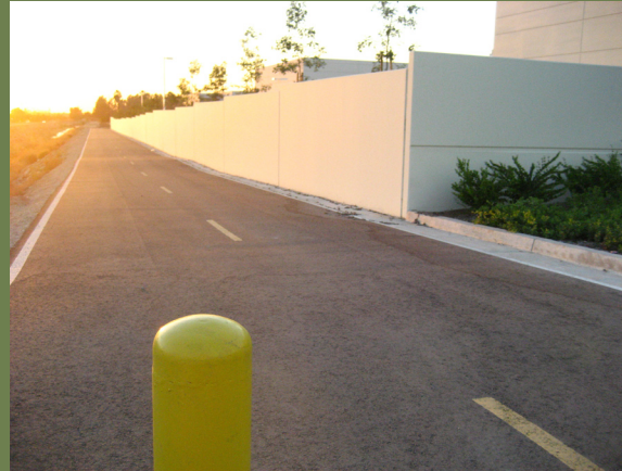
Existing Zanja Creek Trail at Iowa St. facing west
