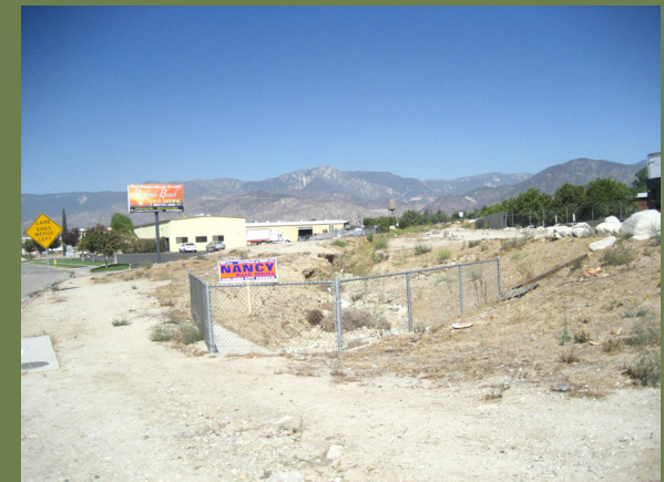
Continuation of abandoned rail corridor and drainage channel north east of Crafton Park facing northeast
