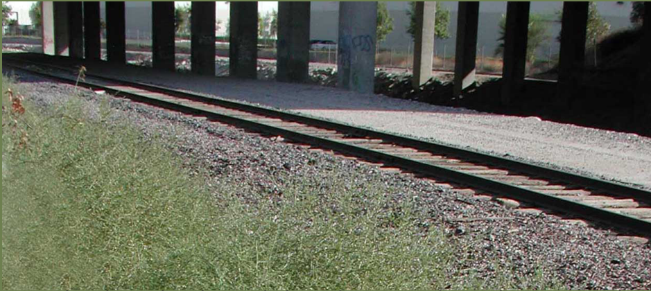
Magnolia Channel and Metrolink tracks passing beneath I-10, viewed from downstream.
