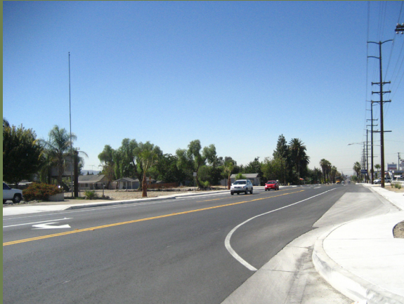
Intersection of Opal Ave. and Wabash Ave. facing southwest toward MWD easement
