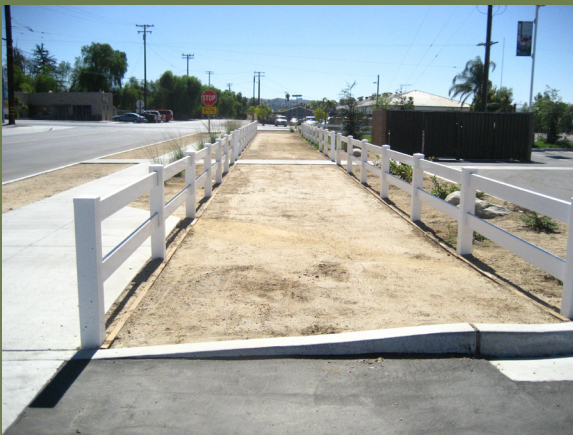
Existing equestrian pathway at the Mentone Sr. Center/Library extending from the intersection of Opal Ave. and Mentone Blvd. north and terminating about 150 feet north of the the Sr. Center/Library
