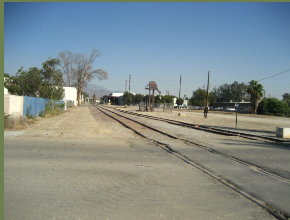
Metrolink tracks at 7th St. facing east toward 9th St.
