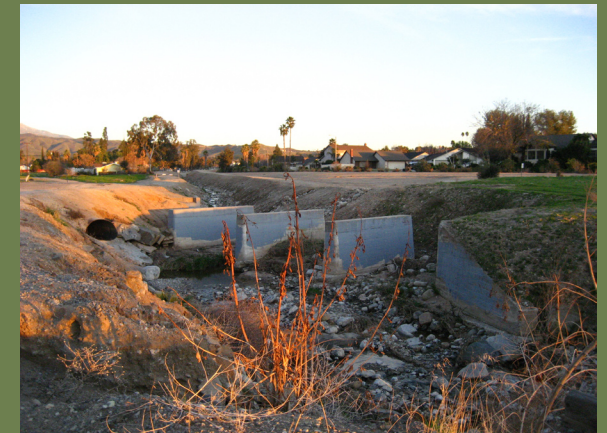
Confluence of Zanja Creek (distant center and foreground), drainage channel inlet (left) and abandoned corridor crossing (right) - facing east
