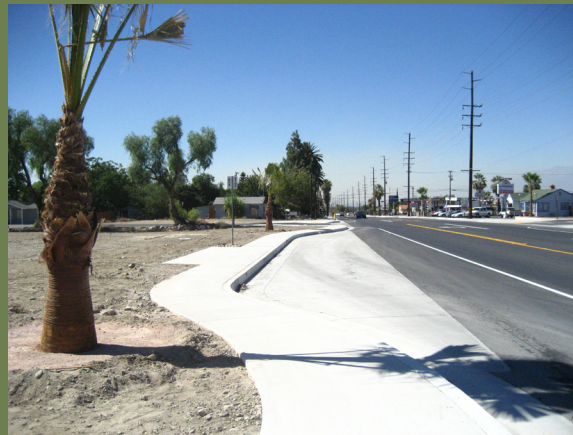
MWD easement at Mentone Blvd. facing west
