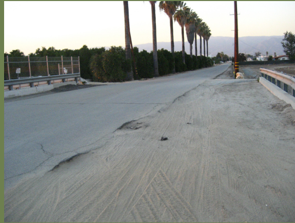
Zanja Creek at Nevada St. facing north
