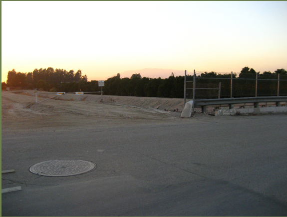
Zanja Creek at Nevada St. facing west
