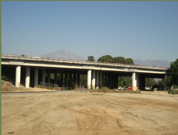
Metrolink tracks at I-10 facing east toward Sylvan Park
