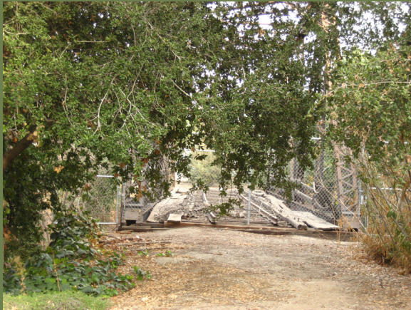
Existing Historic Railroad Bridge at Texas St. and Redlands Blvd.
