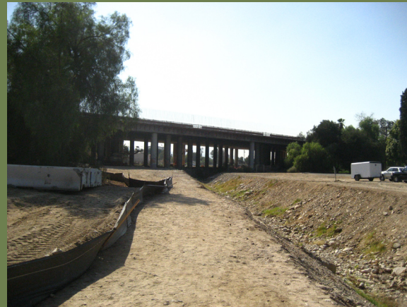
Metrolink tracks at Sylvan Park facing west toward Church St.
