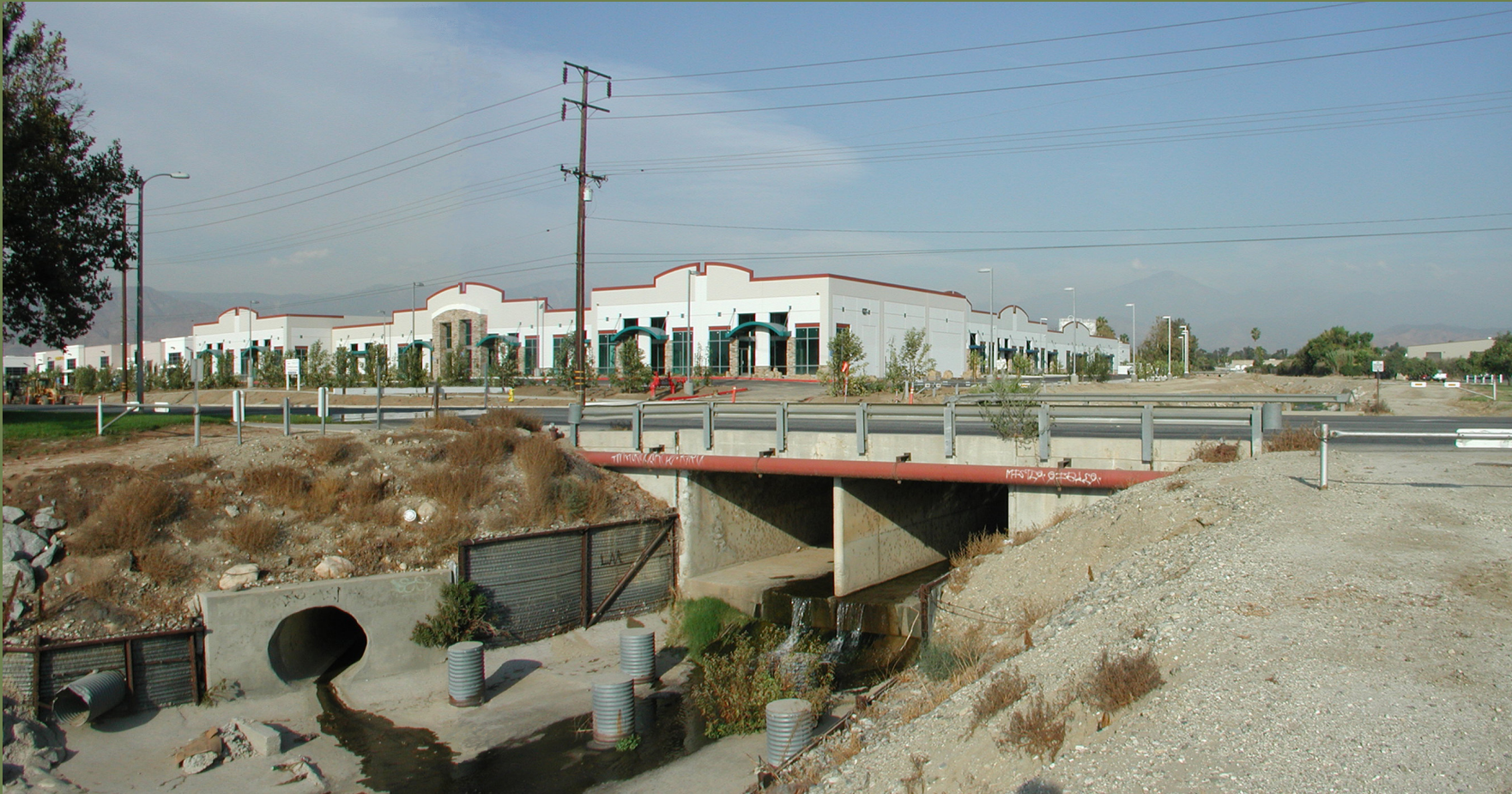
Zanja Creek at Alabama St. looking east
