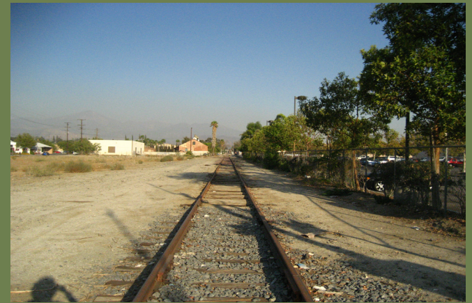
Metrolink tracks at Eureka St. facing east
