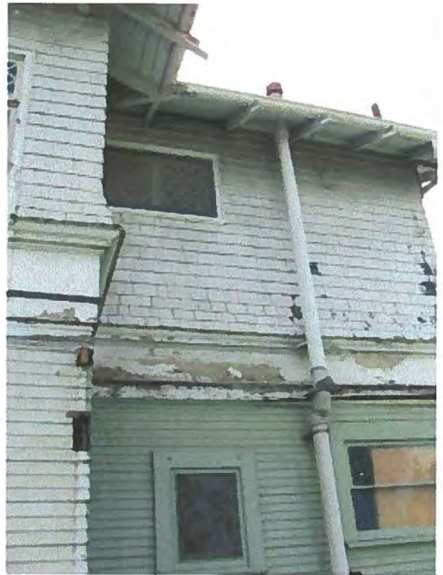
West rear of house
