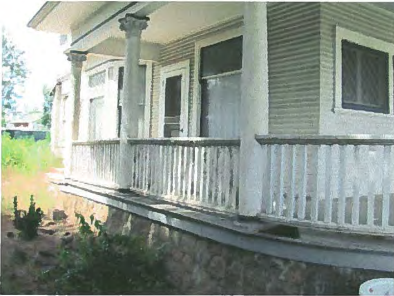
East side; original rock foundation
