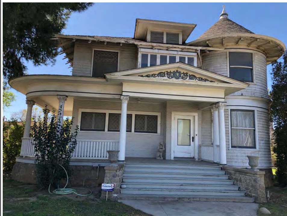
P5a. Front (North) View
