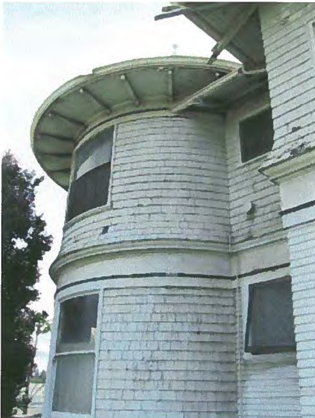
Tower with rafters
