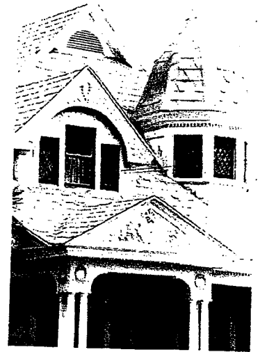
The steep gables create an interesting pattern in themselves. The turret offers a contrasting pattern that is part of the Victorian style. The carved relief trim and different shingles add texture.
