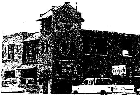
OOPS! An outstanding brick commercial building that has been stuccoed and transformed into a Spanish Colonial Revival.
