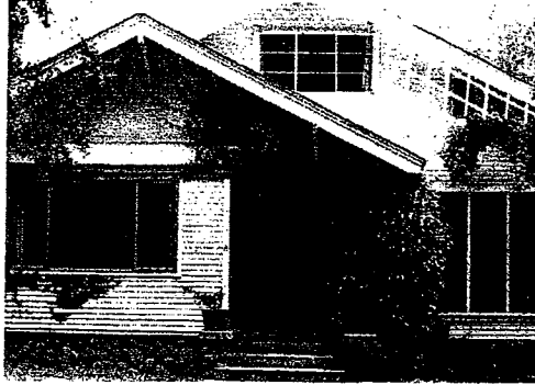
OOPS! Charming original windows and front door almost ruined by new window additions.
