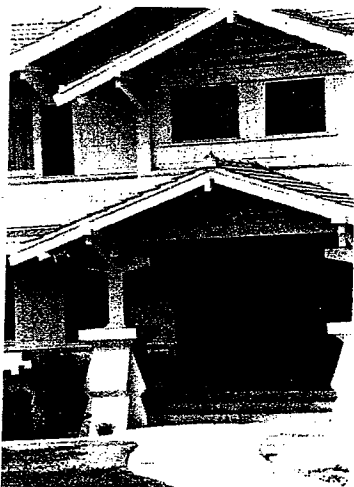
Shingles, tile, elaborate porch piers, create interesting texture. The superimposed gables create the bungalow pattern.
