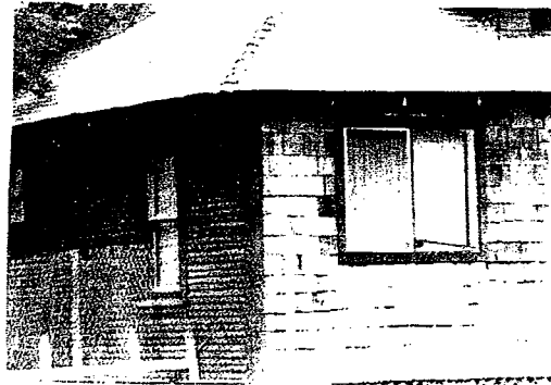
OOPS! The horizontal aluminum windows are incompatible with the original vertical rectangular windows.
