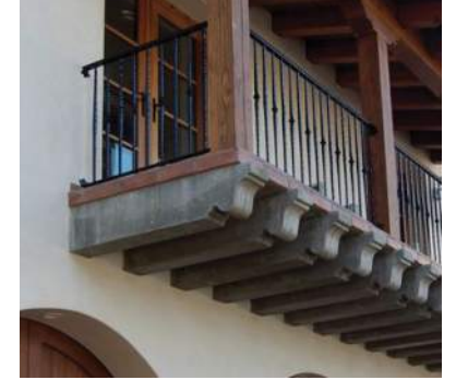
WOOD BEAM BALCONY
