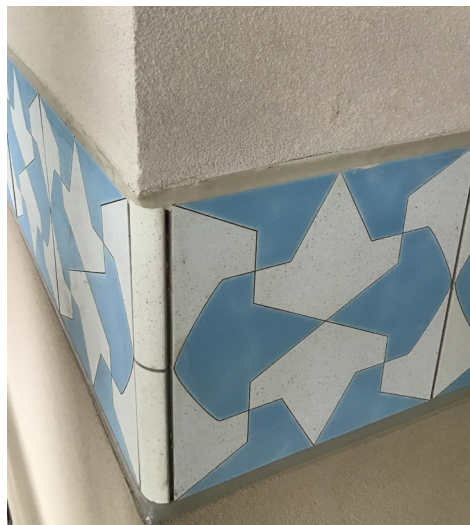
FLUSH TILE DETAILING
