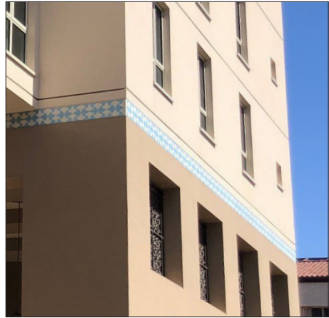
FLUSH TILE DETAILING AT STUCCO
