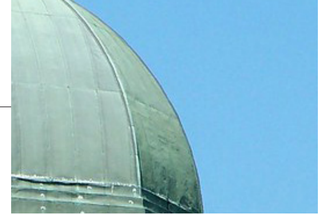
OXIDIZED COPPER SHEET DOME
