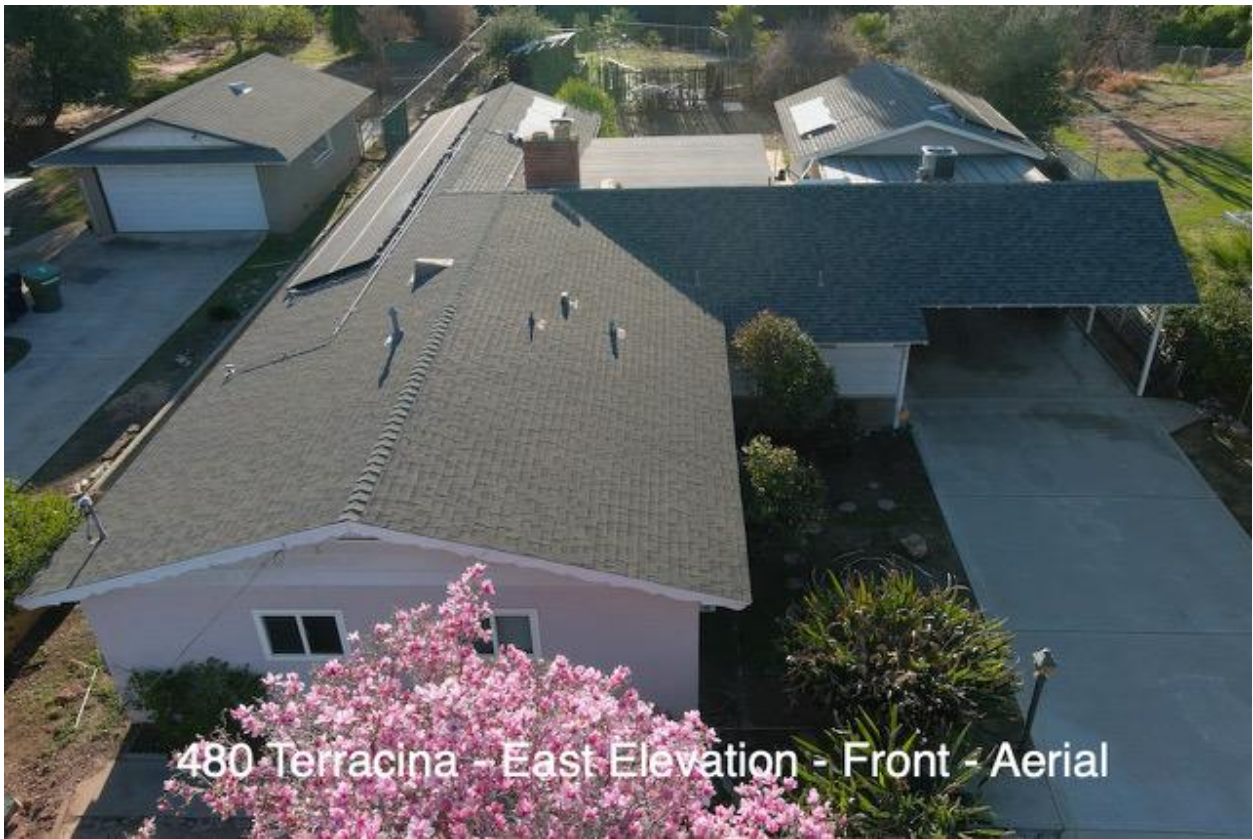
480 Terracina - East Elevation - Front
