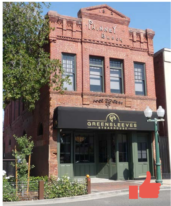
An example of a compatible contemporary awning on a historic building.
