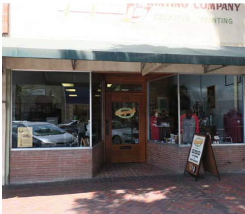
Preserve a historic storefront's relationship to the public right-of-way.
