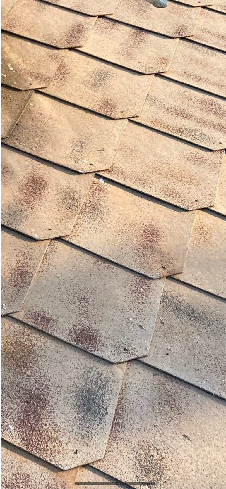
Existing Roofing Material - Photograph
