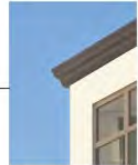
SHEET METAL CORNICE
