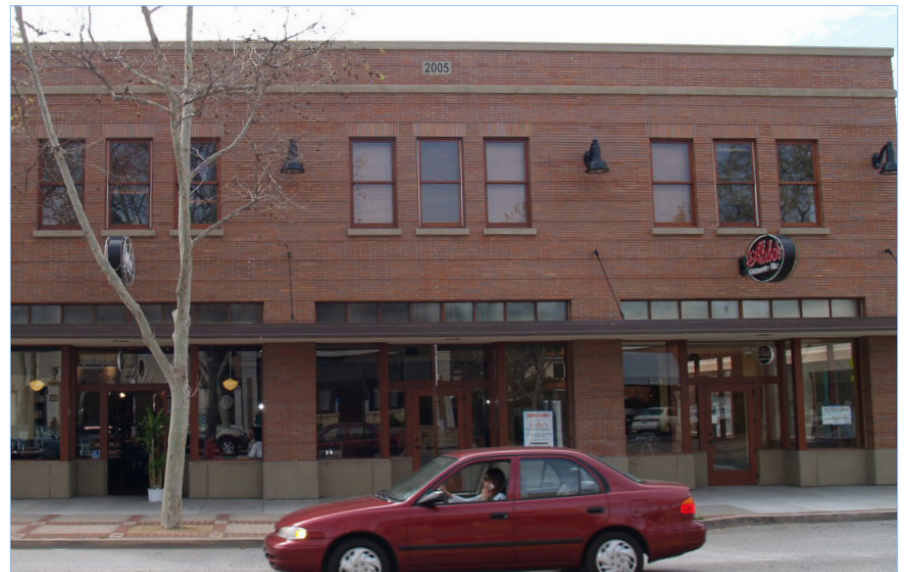
The windows of this mixed-use building are composed according to a logical order. The second floor windows are grouped in threes and centered above the ground floor storefront doors and windows.
