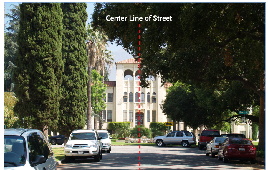
A tower that is placed on the center line of the street.
