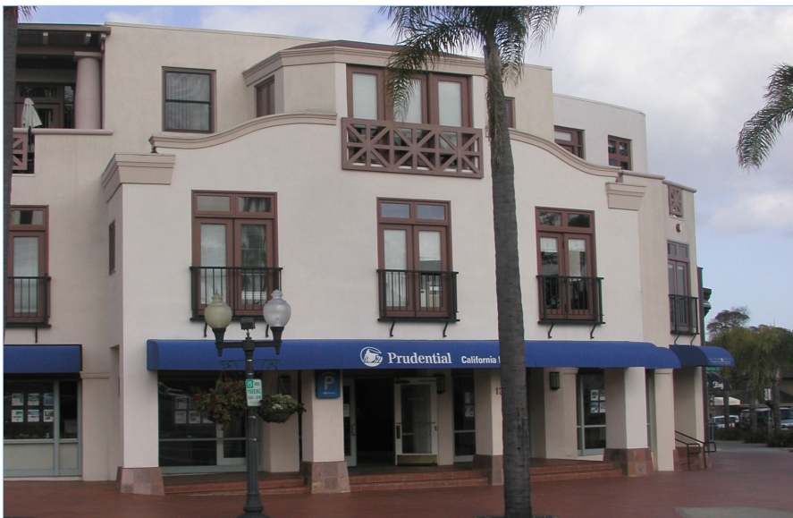
A mixed-use building clad in plaster. The moldings and column bases are constructed of durable materials (precast concrete and tile, respectively).
