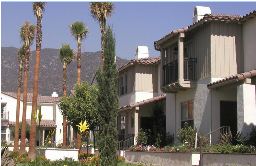
A multi-family building clad in plaster and fiber-cement siding. The vertical transition between the plaster and siding occurs at the inside corners.
