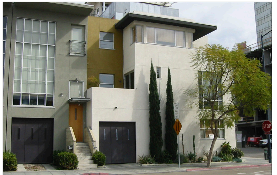
The windows of this rowhouse building are designed to reflect the character and size of the rooms to which they belong: larger windows for formal rooms and smaller windows for bedrooms and bathrooms.
