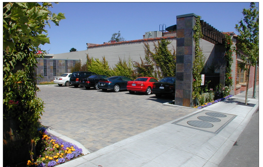
A commercial parking lot that includes planting areas and semi-permeable paving to facilitate rainwater recharging.
