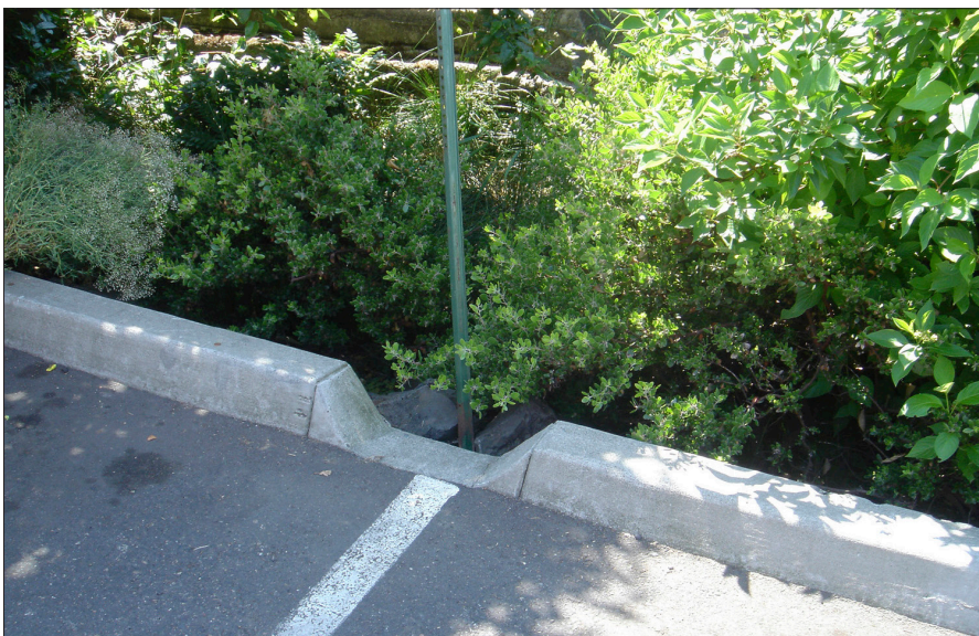
A Low Impact Design strategy whereby a break in the curb allows water to flow into planters.
