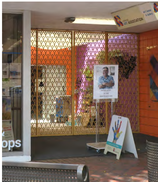
Decorative metal gates at entrance.
