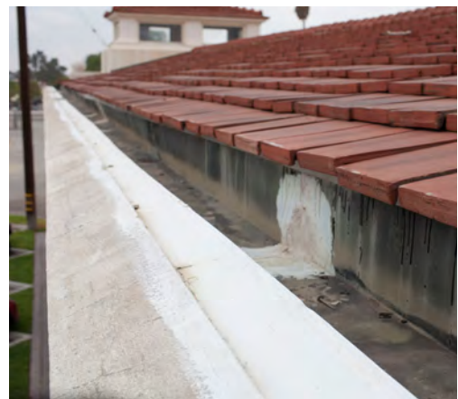
Integral gutter at Santa Fe Depot.
