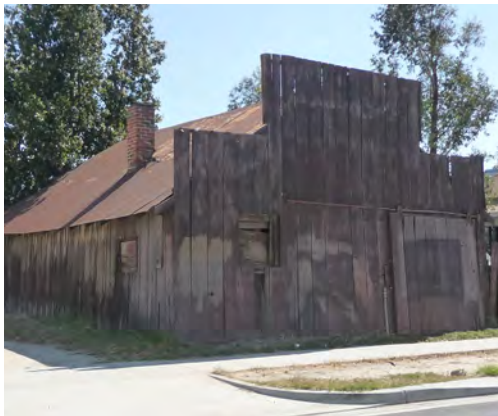
Vertical board cladding on a ca. 1908 blacksmith shop.
