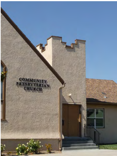
Textured stucco on a Redlands church.
