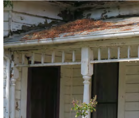
Remove debris from roofs and gutters.
