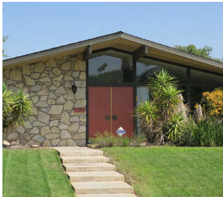
The tall wood doors and clerestory windows on this Contemporary Ranch house are integral to its character.
