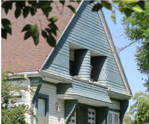
Wood shingle wall cladding.
