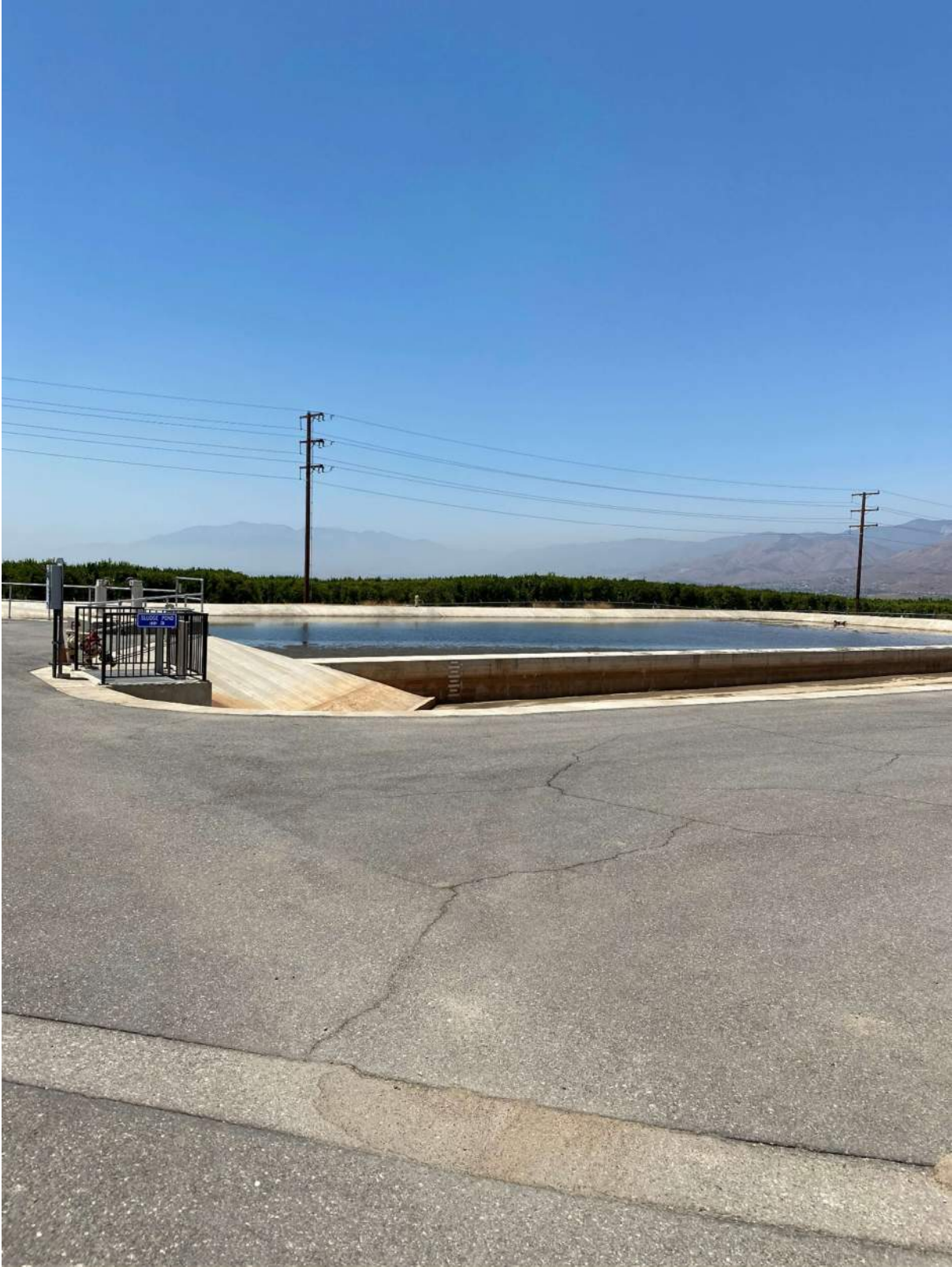
Figure 11 Hinckley WTP Filter Backwash Basin
