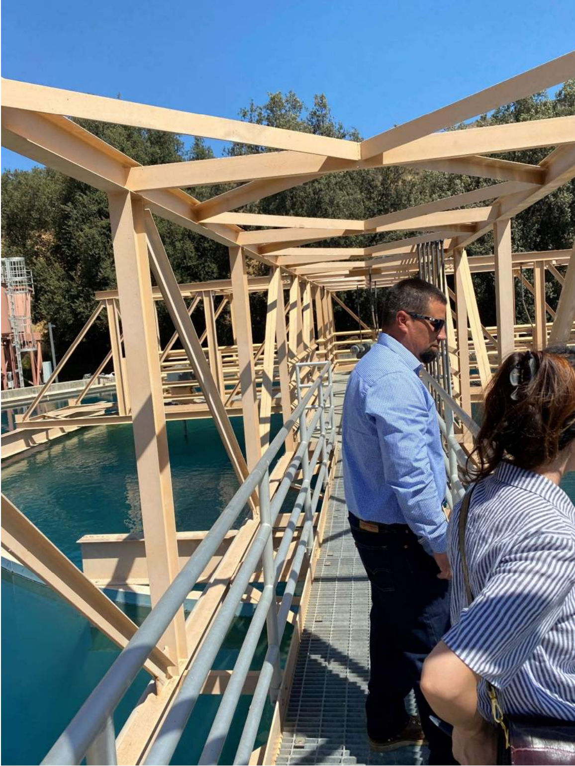
Figure 36 Eimco Settler (Signs of Aging and Corrosion of Mechanical Equipment)
