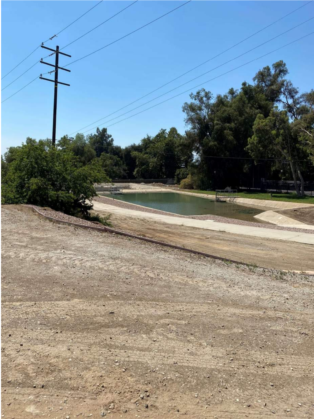
Figure 40 Washwater Reservoir (seems to be in excellent working condition)
