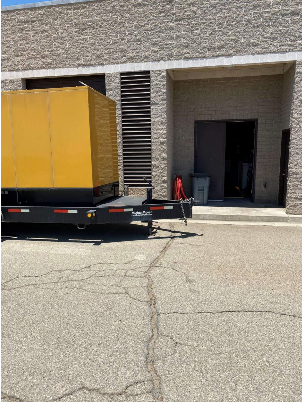
Figure 12 Hinckley WTP Generator Building
