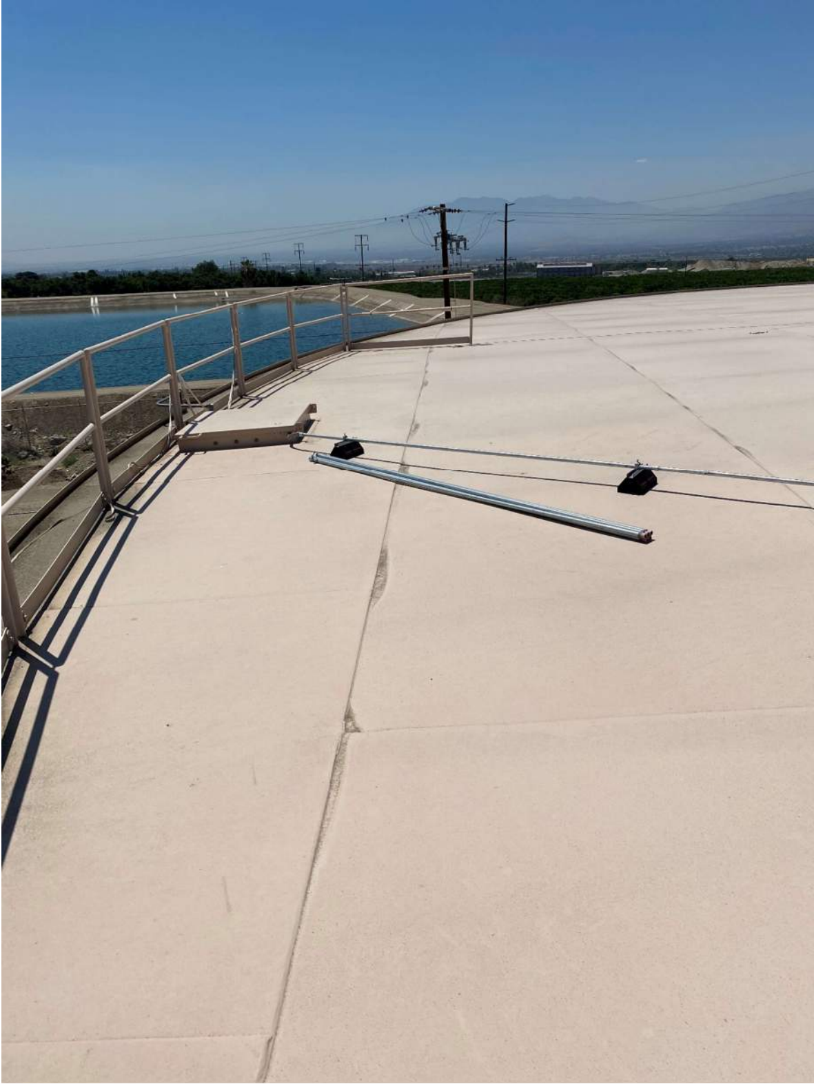
Figure 17 Agate Reservoir Roof
