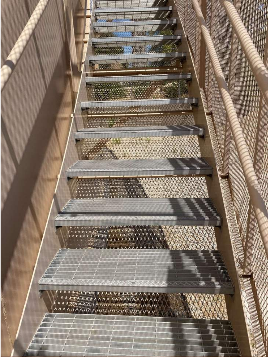
Figure 18 Agate Access Stairway with Partial Enclosure Safety Cage
