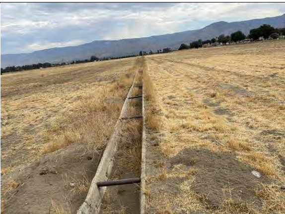
View of concrete lined former irrigation channel
