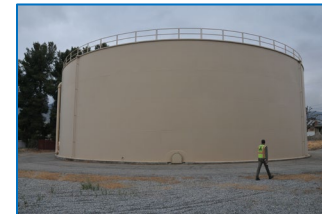
Ward Way Reservoir
