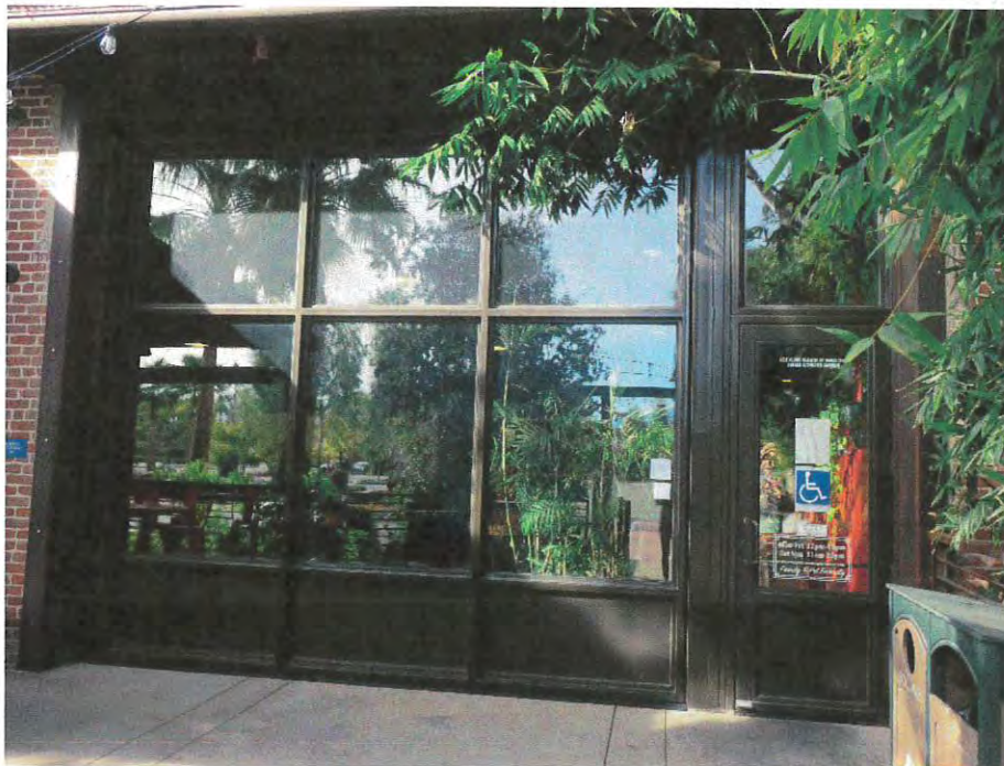
Photo 12 Close-up of the new tilt-up steel door assembly at the north end of the east façade.
