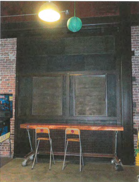
Photo 20 Interior close-up of the new zinc paneled door.
