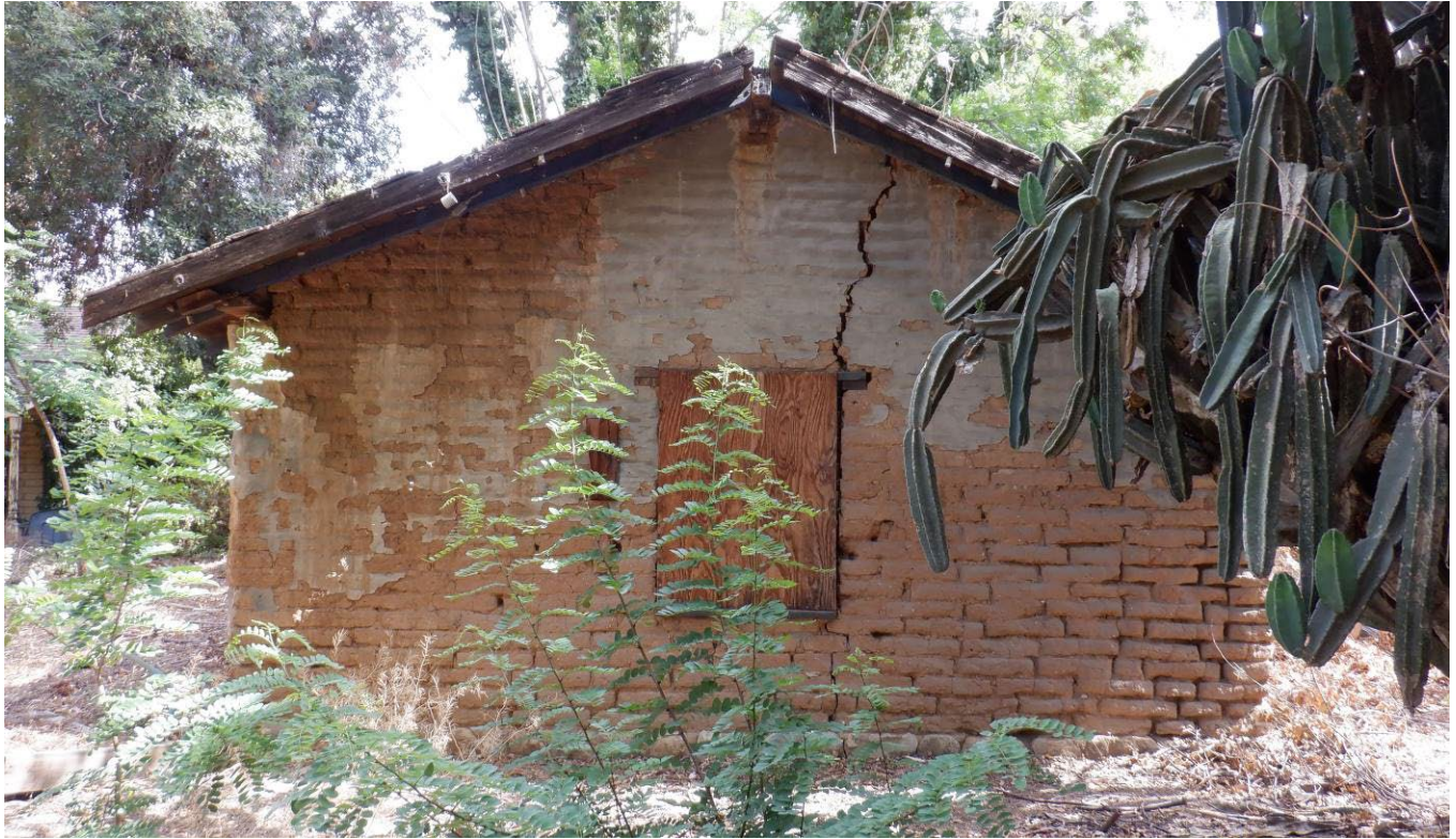
South elevation detail. View north. (Michael Baker International, June 22, 2022)
