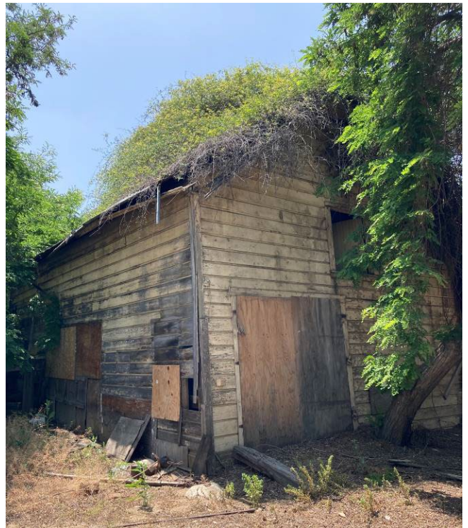
Barn building (Monte LLC, May 3, 2022)
