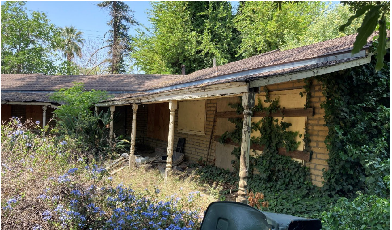
Detail of the porch on residence. View northwest. (Monte LLC, May 3, 2022)
