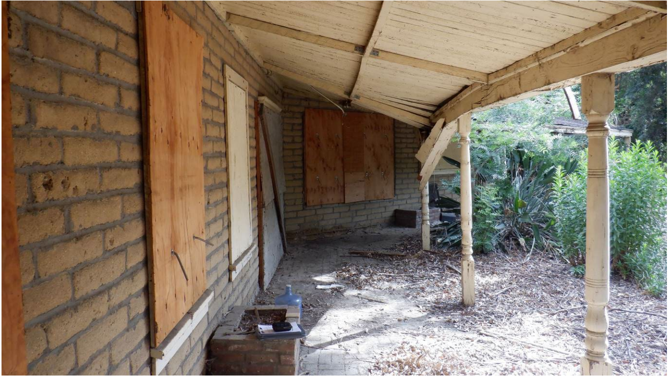
Porch, west wing. View east. (Michael Baker International, June 22, 2022)
