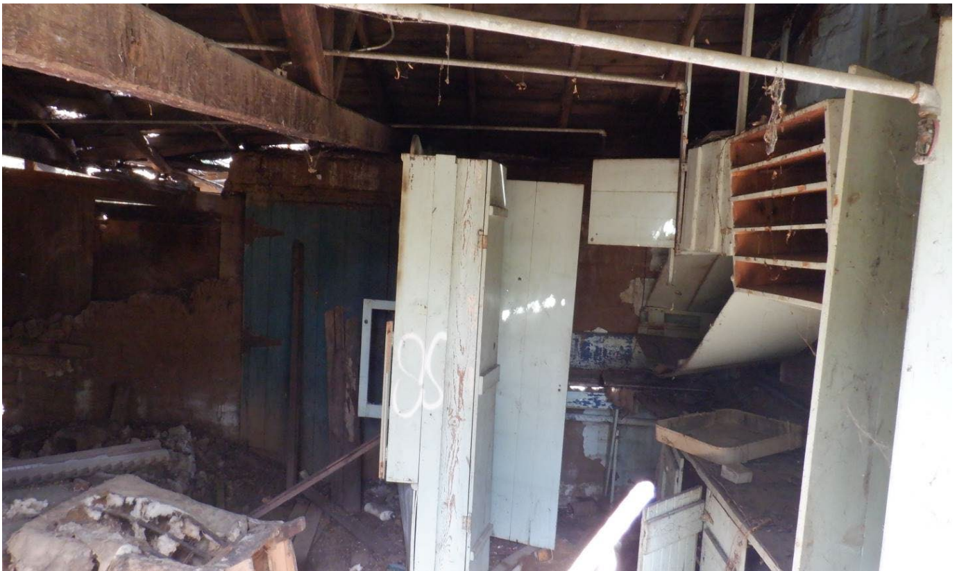
Interior detail of c. 1925 adobe building. (Michael Baker International, June 22, 2022)
