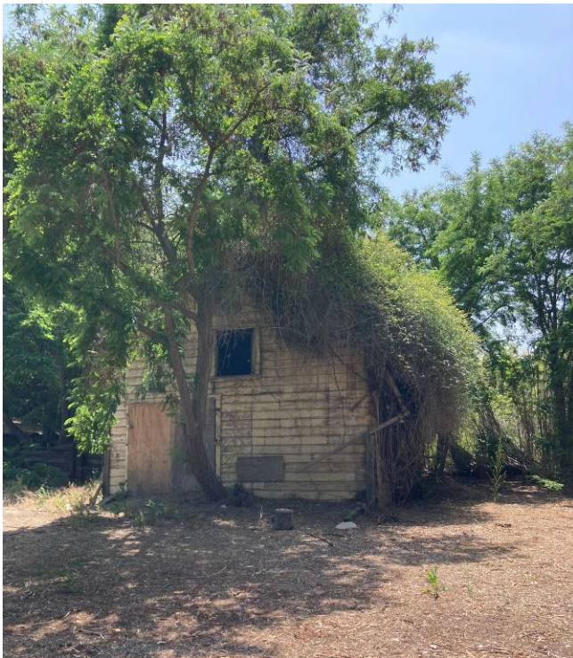
Circa 1925 barn building southeast of residence. View south (Monte LLC, May 3, 2022)
