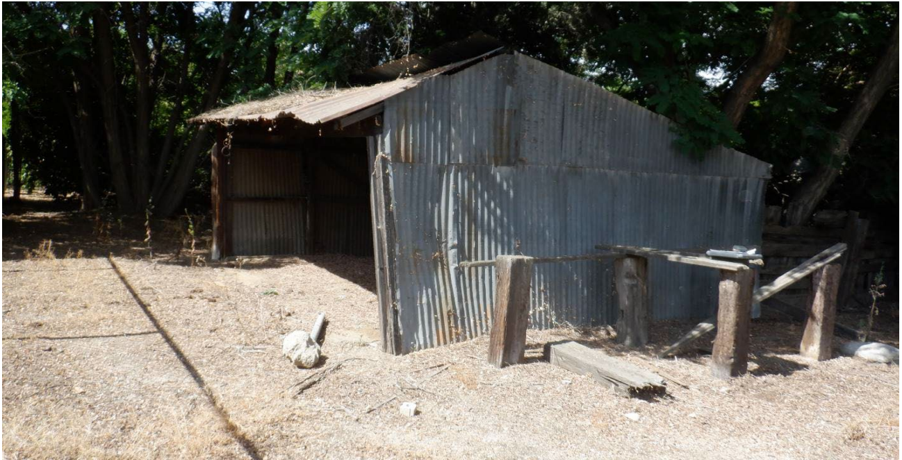
Circa 1960 wood-framed shed with corrugated metal, northeast of wood barn. View southwest. (Michael Baker International, June 22, 2022)
