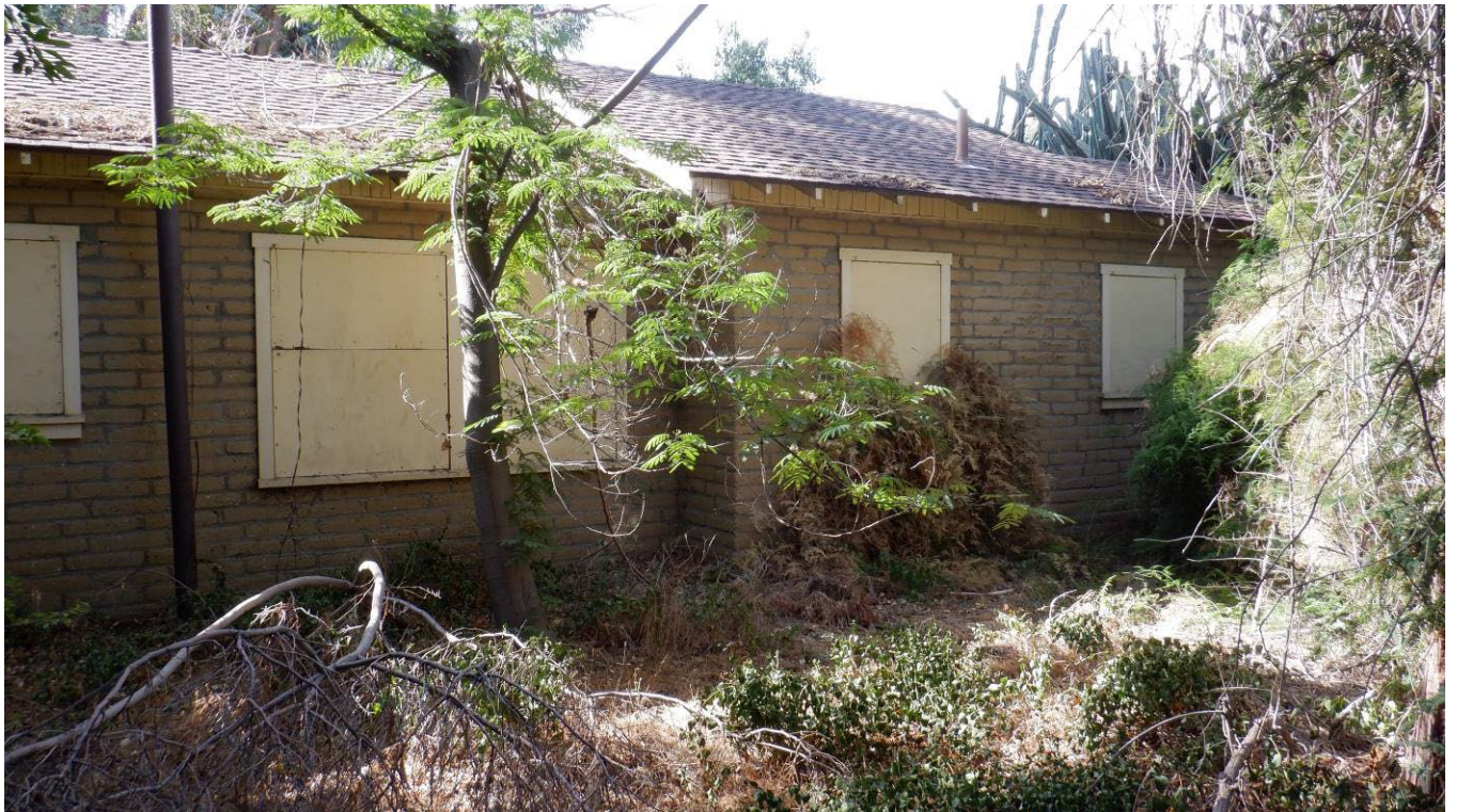
North elevation of residence. View south. (Michael Baker International, June 22, 2022)
