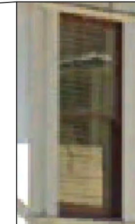
WINDOW & BUILDING TRIM MATERIAL-1/6" PAINTED DOUG. FIR WHITE IN COLOR TO MATCH EXISTING RESIDENCE
