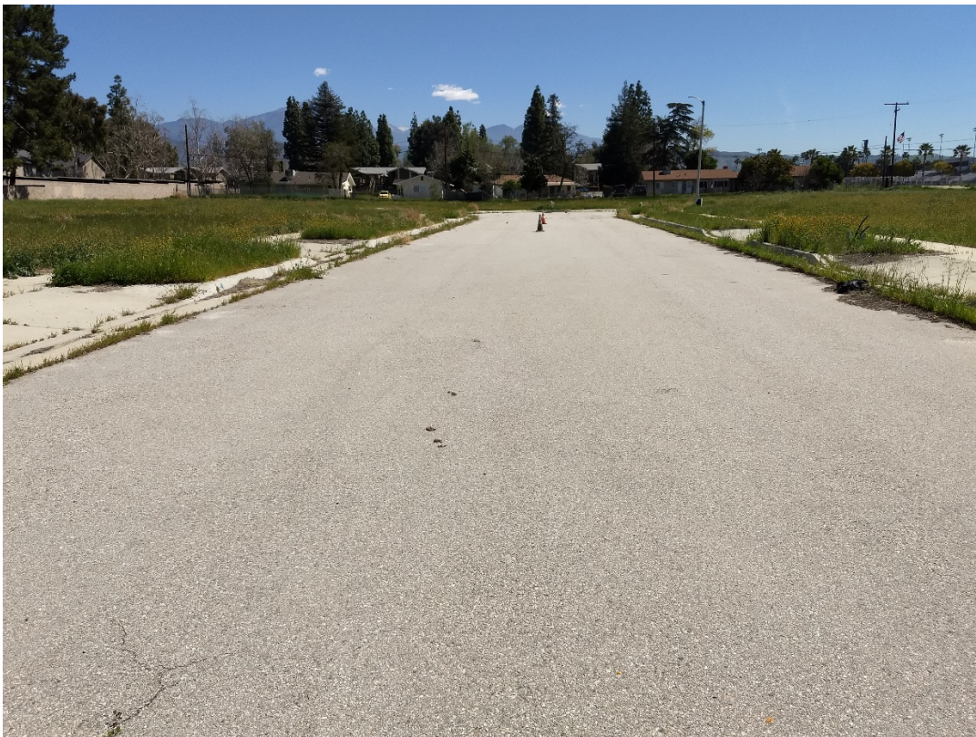
Photograph #4: Existing cul-de-sac and driveway, Looking East
