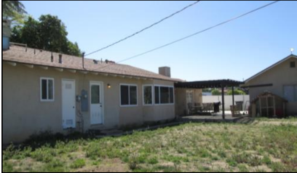
Figure 7: Rear (west) elevation of 1205 North University Street. Unattached two-car garage to the right of the photograph. View looking south.
