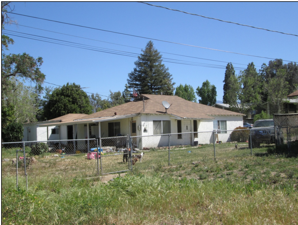
Rear elevation, view looking north-northeast.
