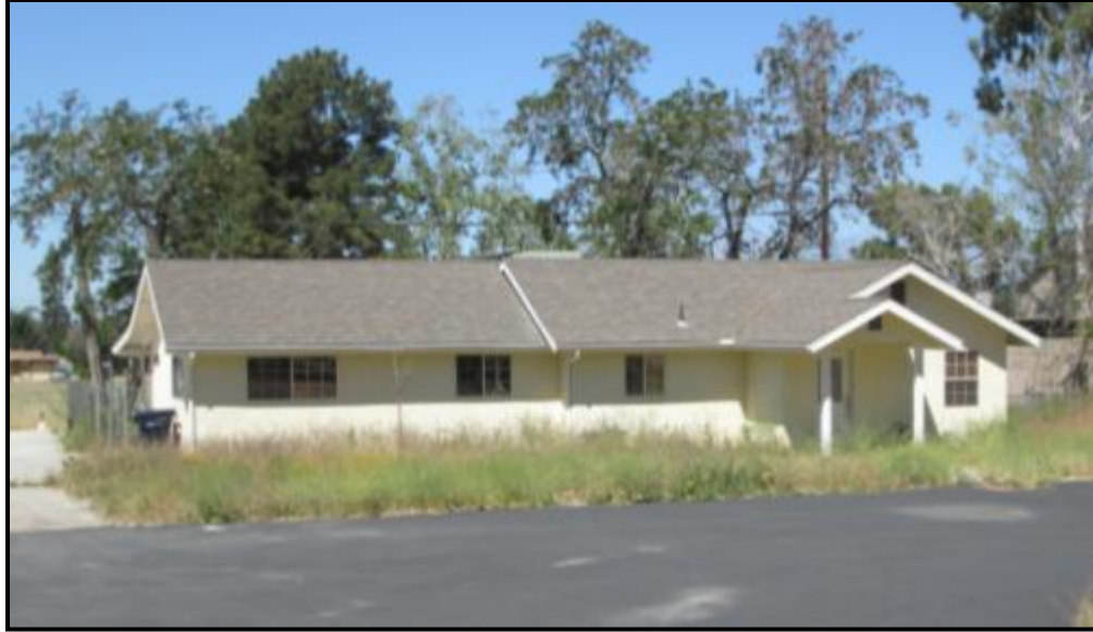
Figure 10: Front elevation of 1219 North University Street. View looking west.
