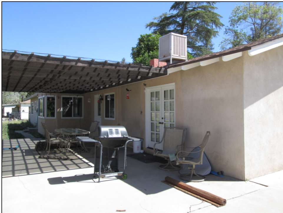
Rear elevation, view looking north.
