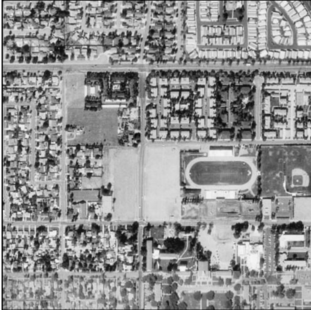
Figure 5: Aerial view of the Redlands University stadium and changes to the surrounding landscape in 1995. (East Lugonia Avenue runs east-west, north of the stadium.)
