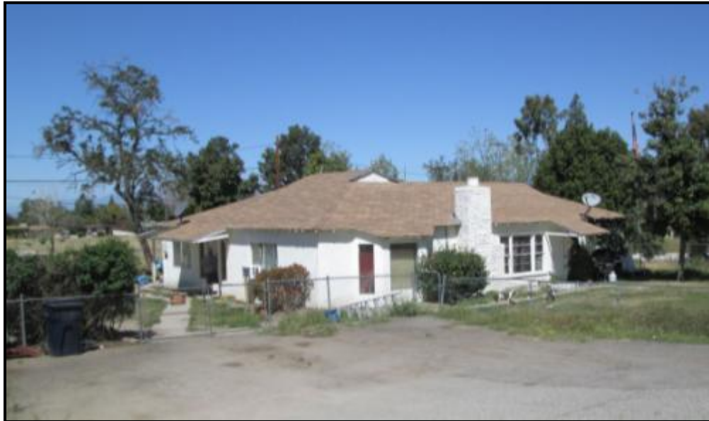
Figure 8: Front elevation of 1215 North University Street. View looking northwest.
