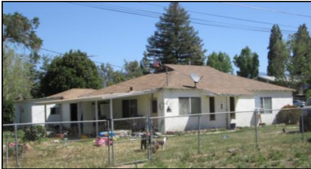
Figure 9: South and rear (west) elevation of 1215 North University Street. View looking northeast.
