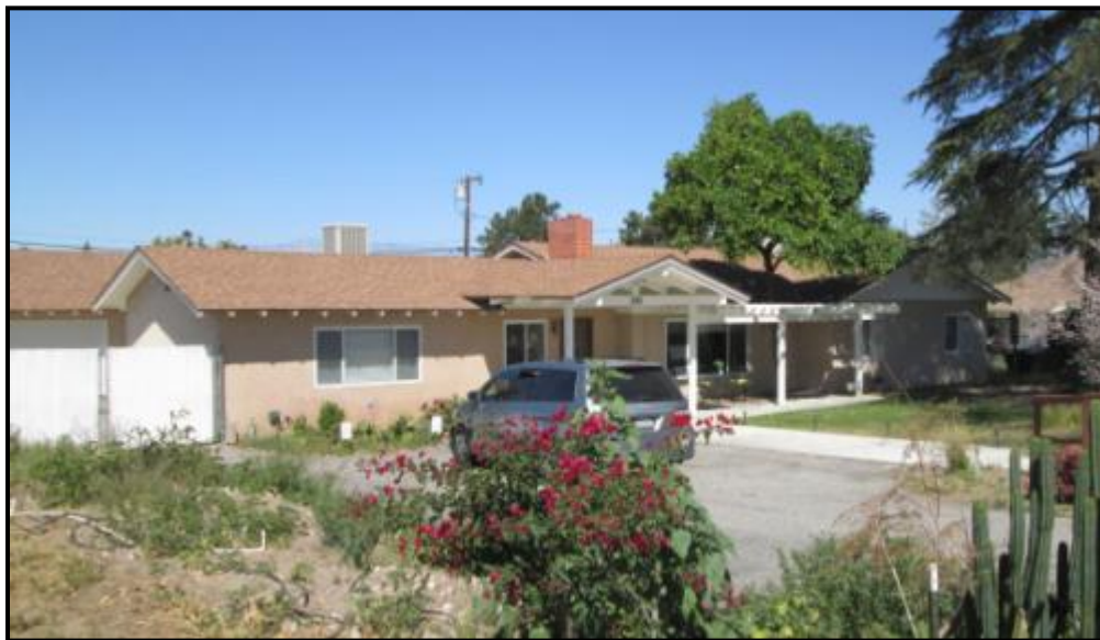
Figure 6: 1205 North University Street, front elevation. View looking northwest.
