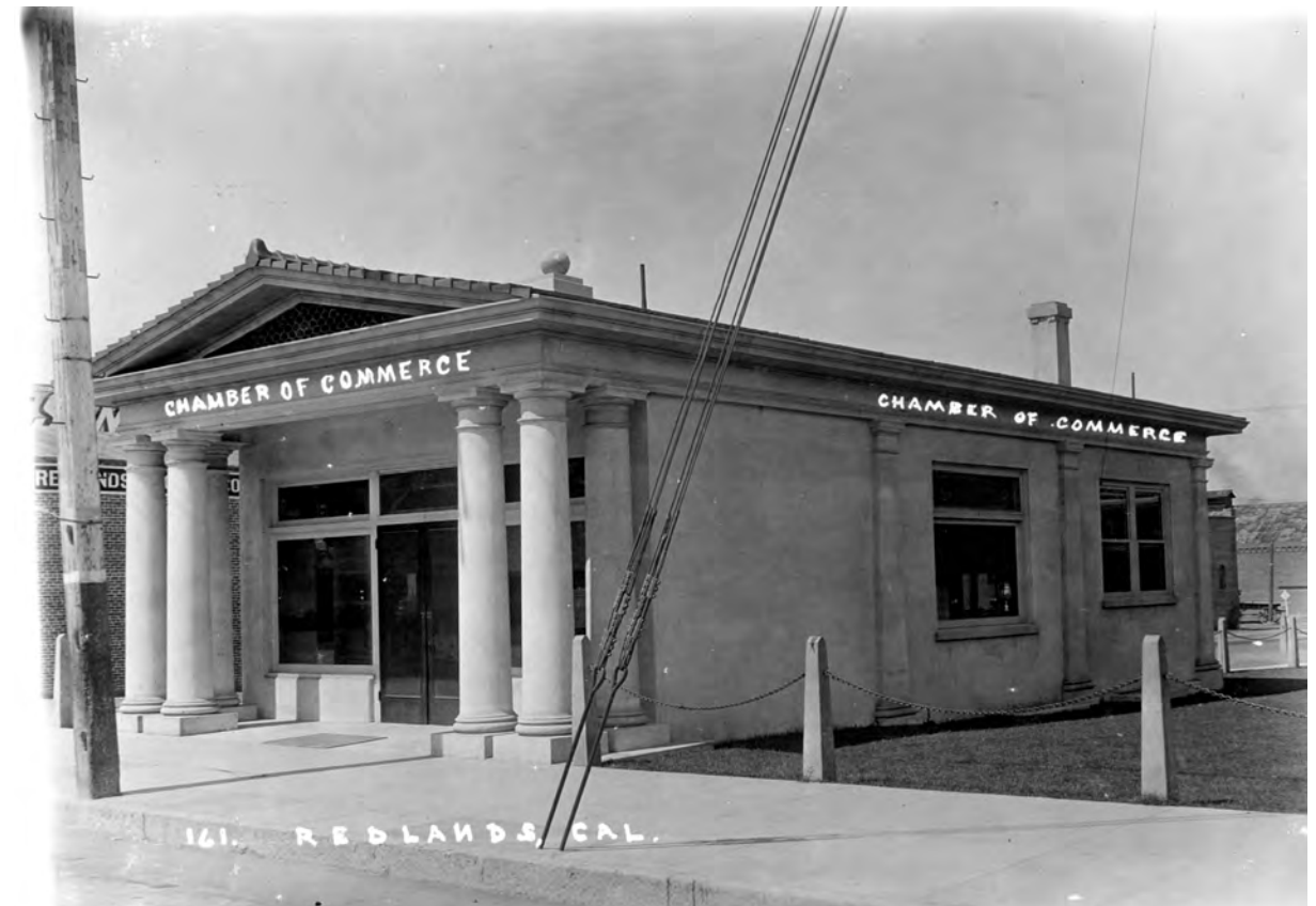
Chamber of Commerce Building, ca. 1915.
