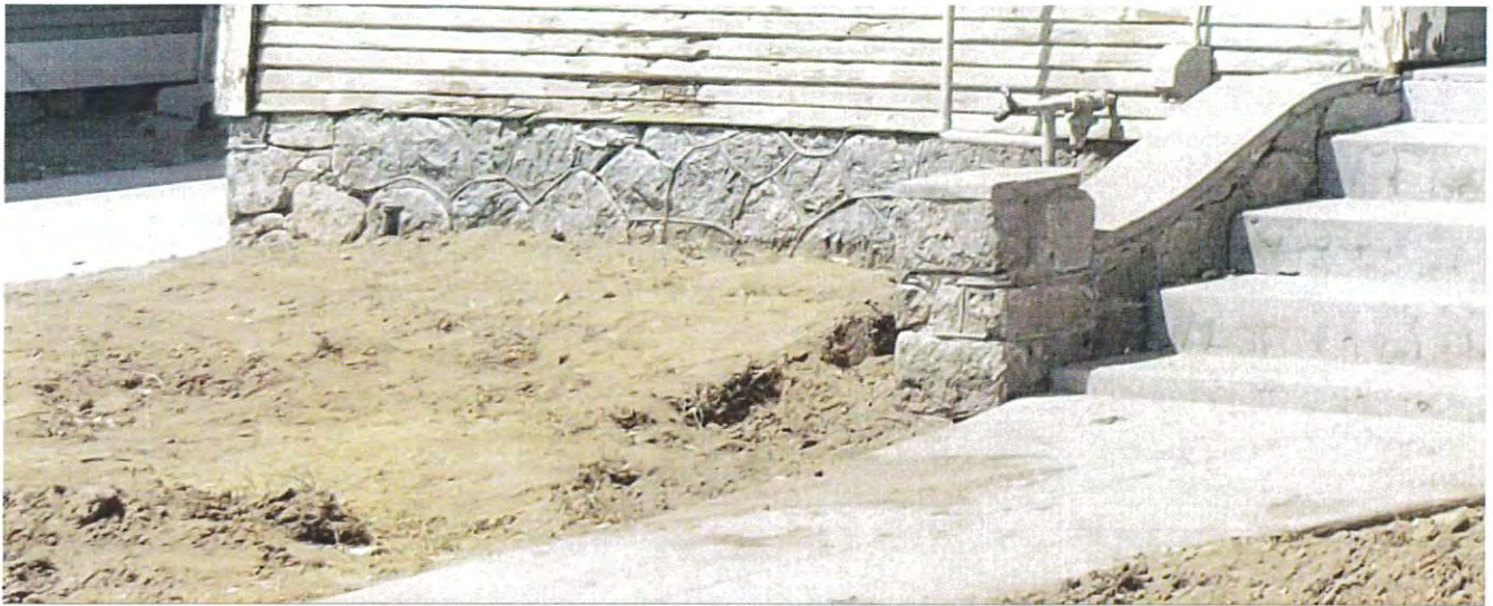
Front (South) Elevation - Image of granite foundation
