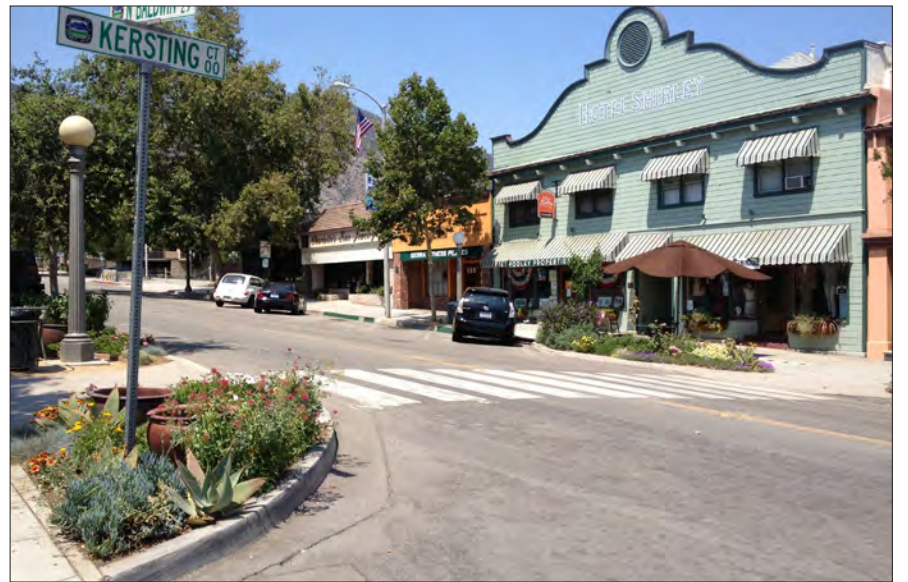
A crosswalk with continental striping, bulb-outs, and drought-tolerant landscaping.
