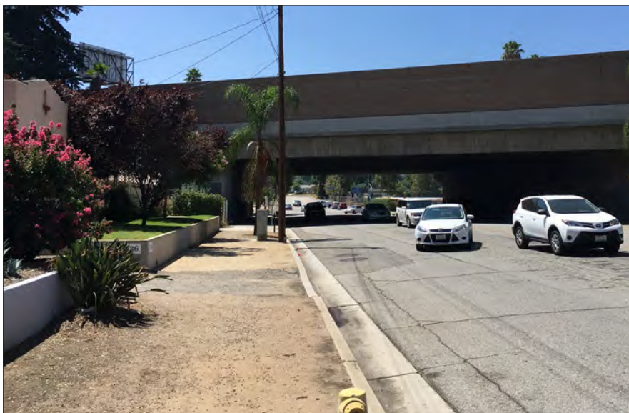
Missing sidewalks along University Street and the inadequately lit freeway underpass.
