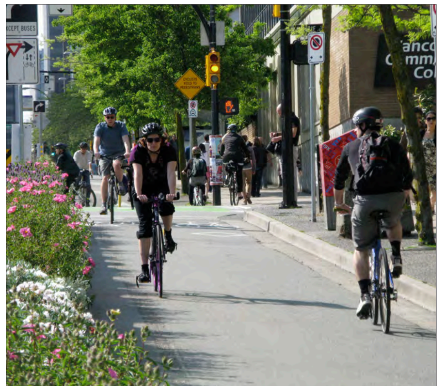
A dedicated bike lane separated from traffic with a planter.
