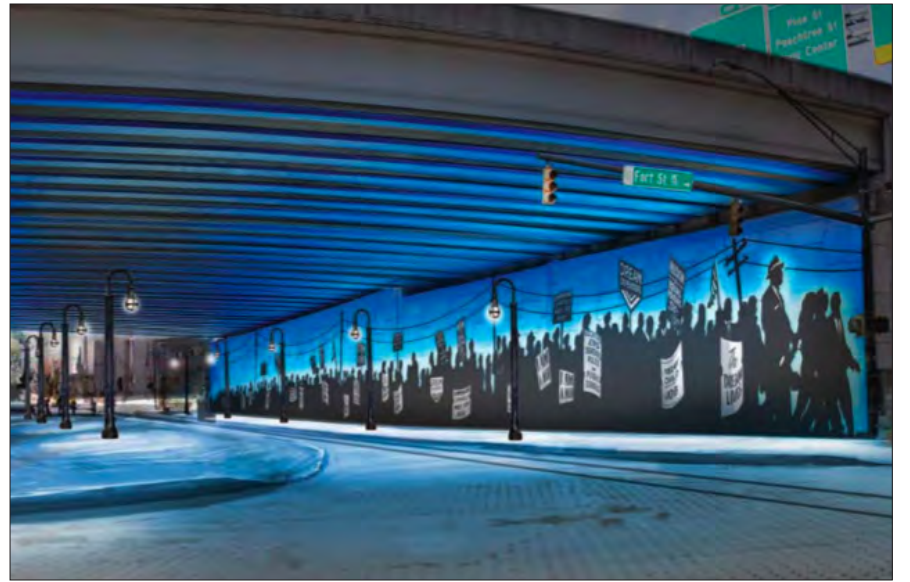
A freeway underpass with creative lighting and artwork.
