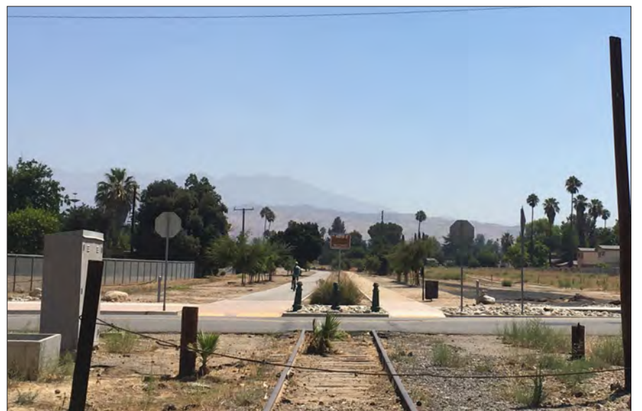
The existing terminus of the Orange Blossom Trail at Grove Street.
