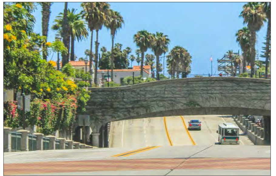
A freeway overpass designed as a traditional bridge. Pedestrian circulation is separated from the roadway by columns and railings.
