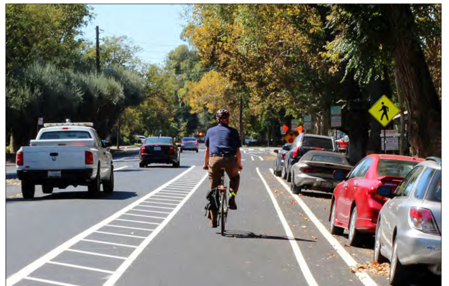
A Class II bike lane is separated from moving and parked cars by painted buffers.
