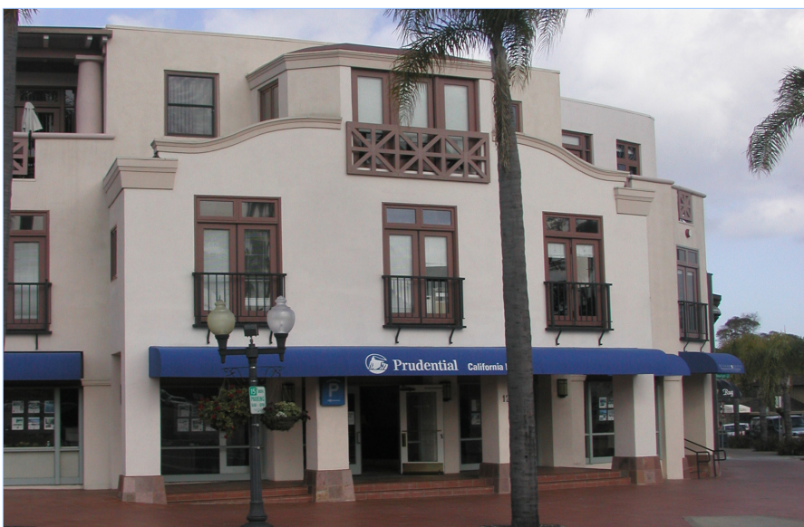
A mixed-use building clad in plaster. The moldings and column bases are constructed of durable materials (precast concrete and tile, respectively).
