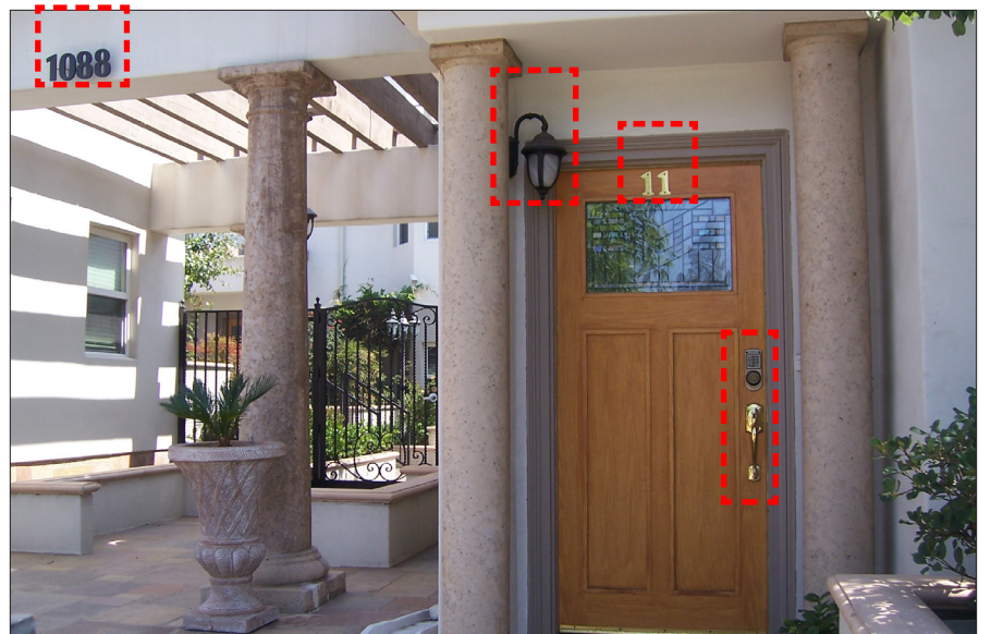
AVOID. Lamps, address signs, and columns are inconsistent in style and finish.
