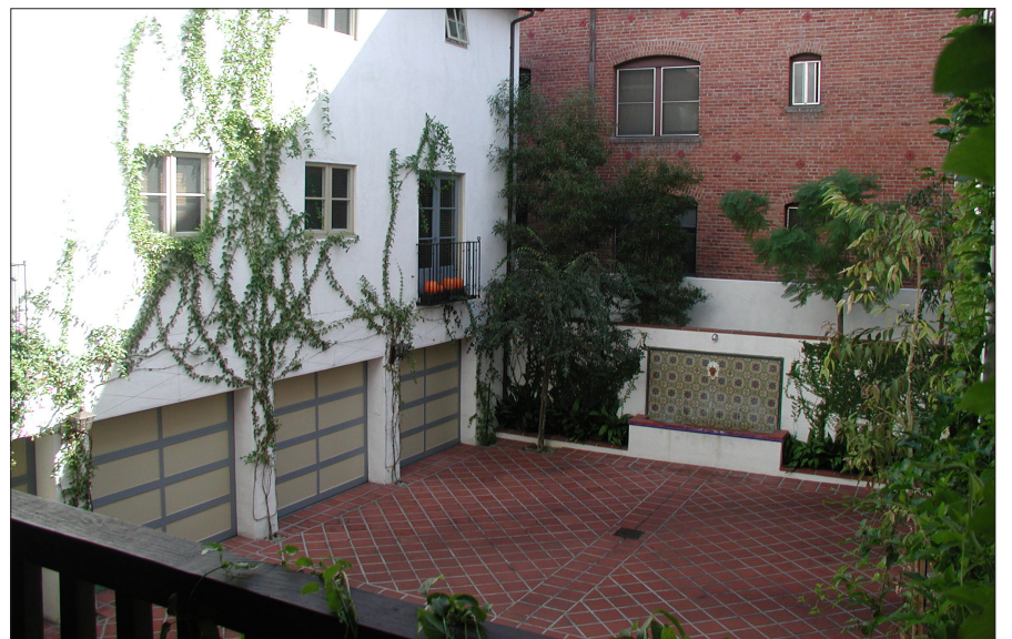
The parking court of a multi-family residential building is paved with terra cotta tiles.
