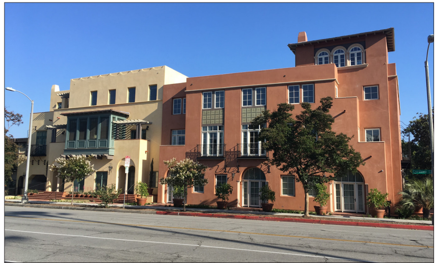
The main volume of this multi-family building is stepped-back from the street. Further articulation is achieved by making the building look like two buildings.
