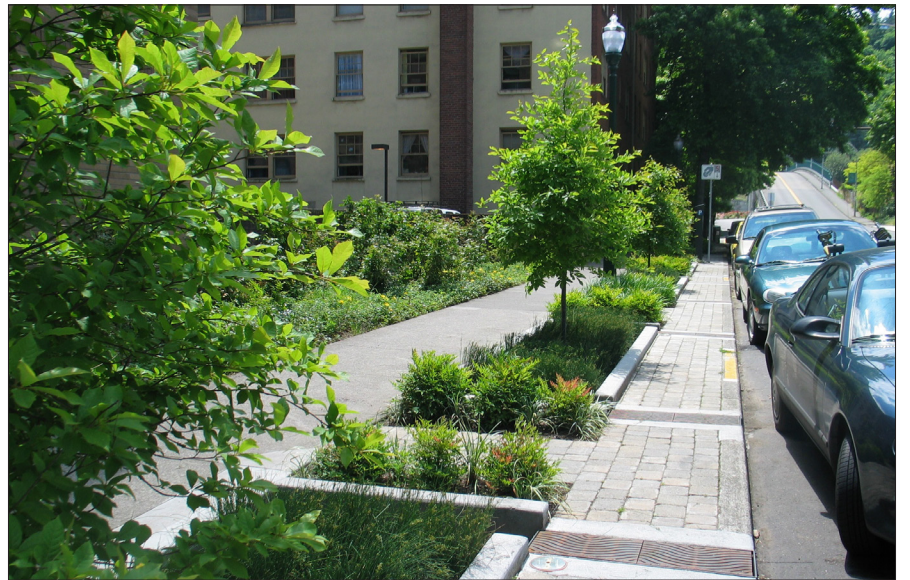
Runoff from the street is directed into planters.
