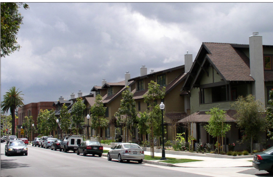
Individual buildings on a site over 150 feet in length designed with varied roof forms and different wall colors.
