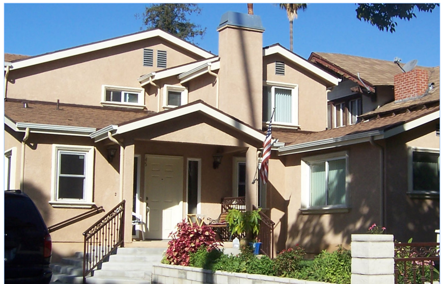
AVOID. Random window placement with windows not relating by shape and proportion to one other.
