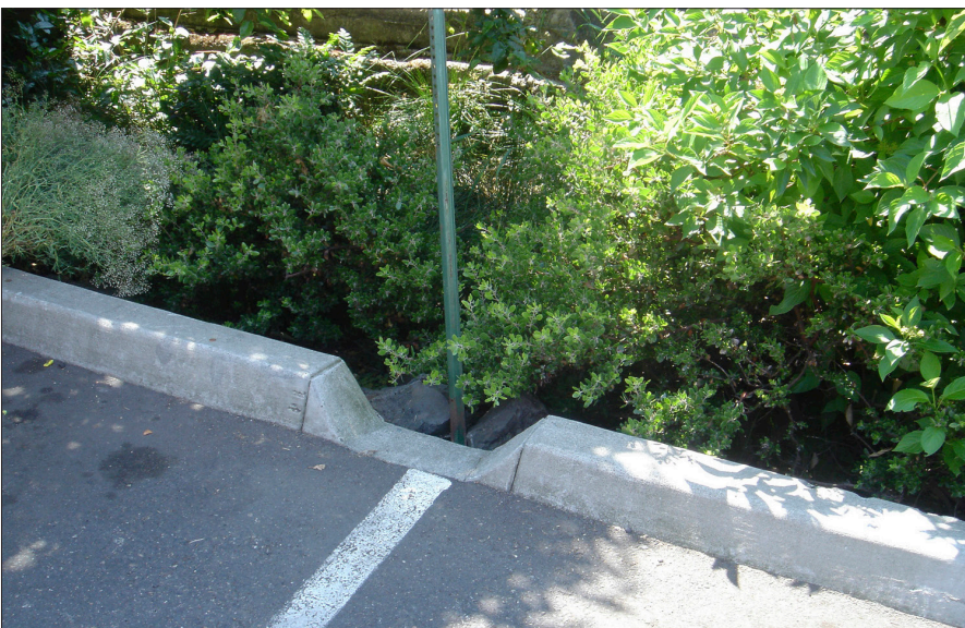
A Low Impact Design strategy whereby a break in the curb allows water to flow into planters.
