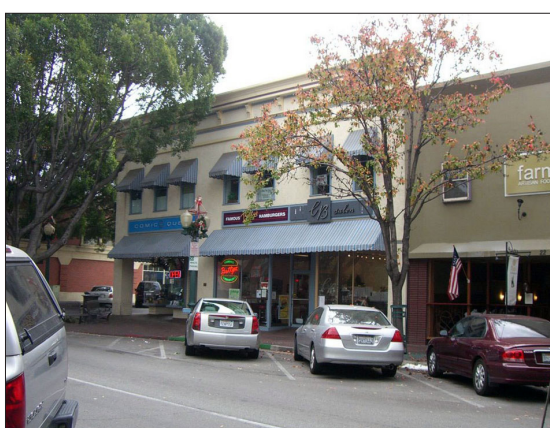
Two-story mixed-use building along State Street.
