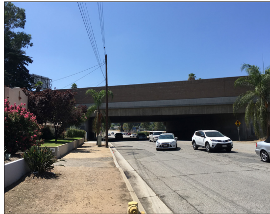
Missing sidewalks and bicycle facilities.
