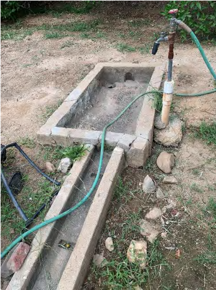
Photograph 3: Detail, gravity-fed irrigation canal connected to a small cement basin at its southeast terminus, July 25, 2019.
