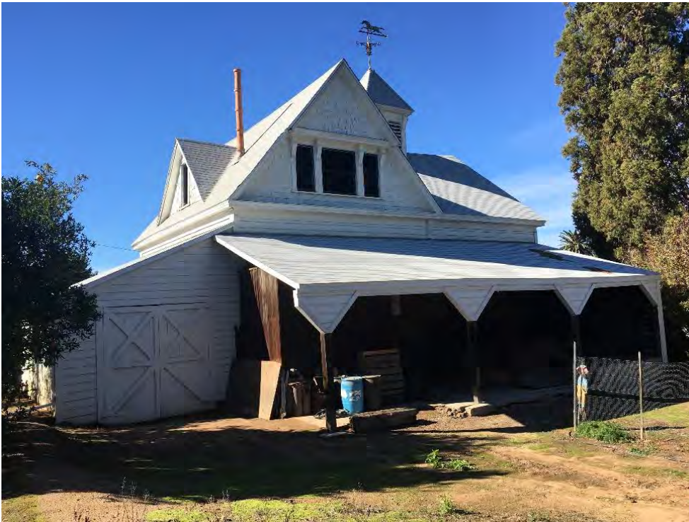
Photograph 4: Northeastern elevation with cover
