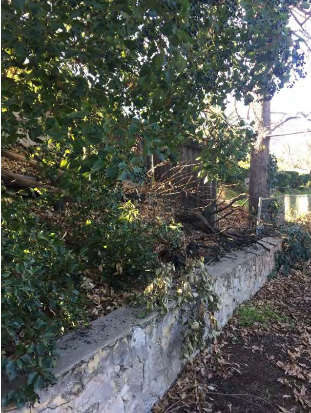
Photograph 2: Detailed view of the concrete masonry footing along the southeast boundary, January 28, 2020.
