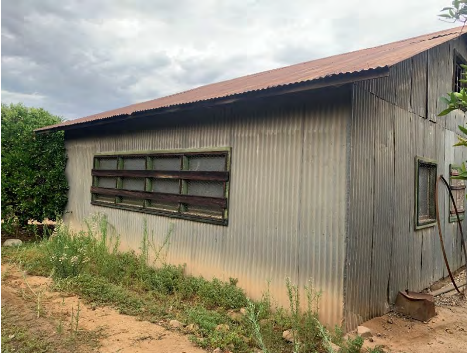
Photograph 4: Southeast and northeast elevations, side windows in view, camera facing west, July 25, 2019.
