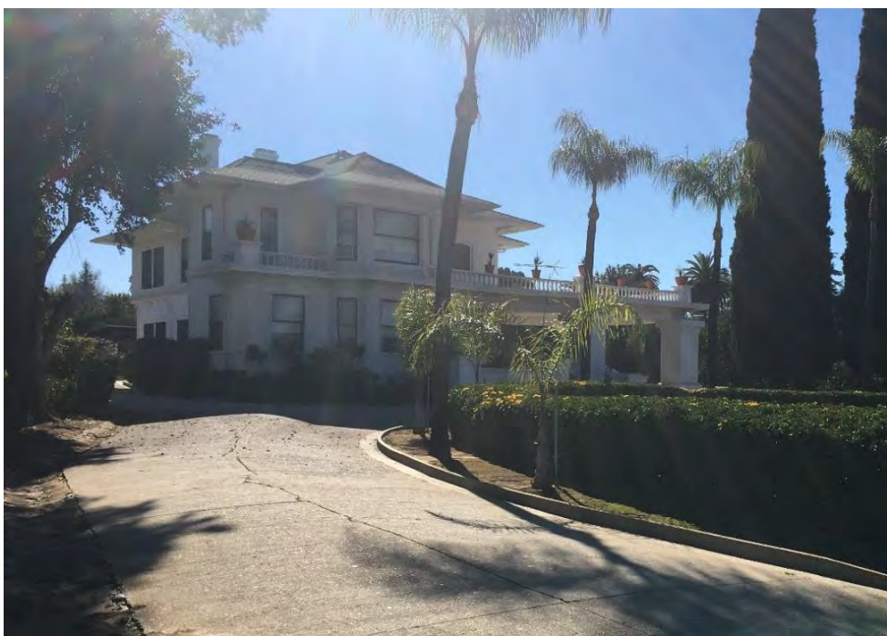
Photograph 3: Northwest and northeast elevations, camera facing south, January 9, 2019.
