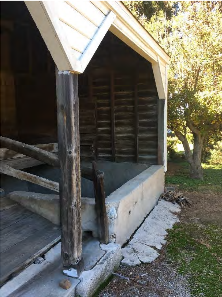
Photograph 6: Cement basin adjacent to wooden entryway in northernmost corner of the carriage house, January 9, 2019.
