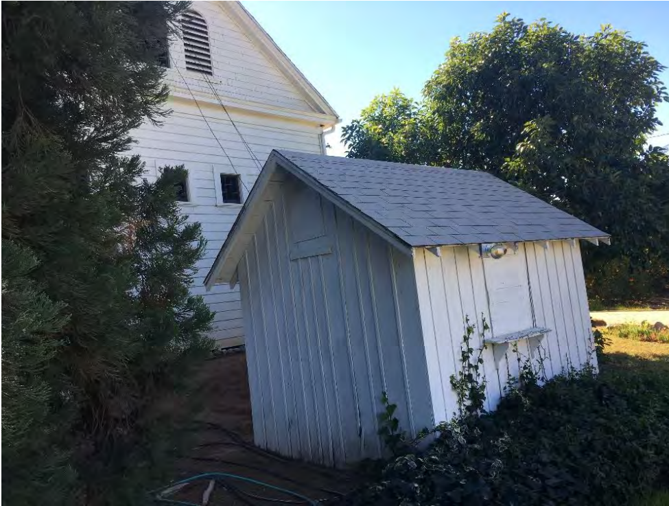
Photograph 9: Northwest and northeast elevations of a small wooden shed located adjacent to the carriage house, northwest elevation of the carriage house visible as well, camera facing south, January 9, 2019.
