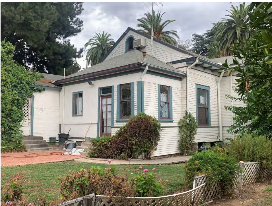
Photograph 11: Northeast and northwest elevations with enclosed back patio also in view, camera facing south, July 25, 2019.
