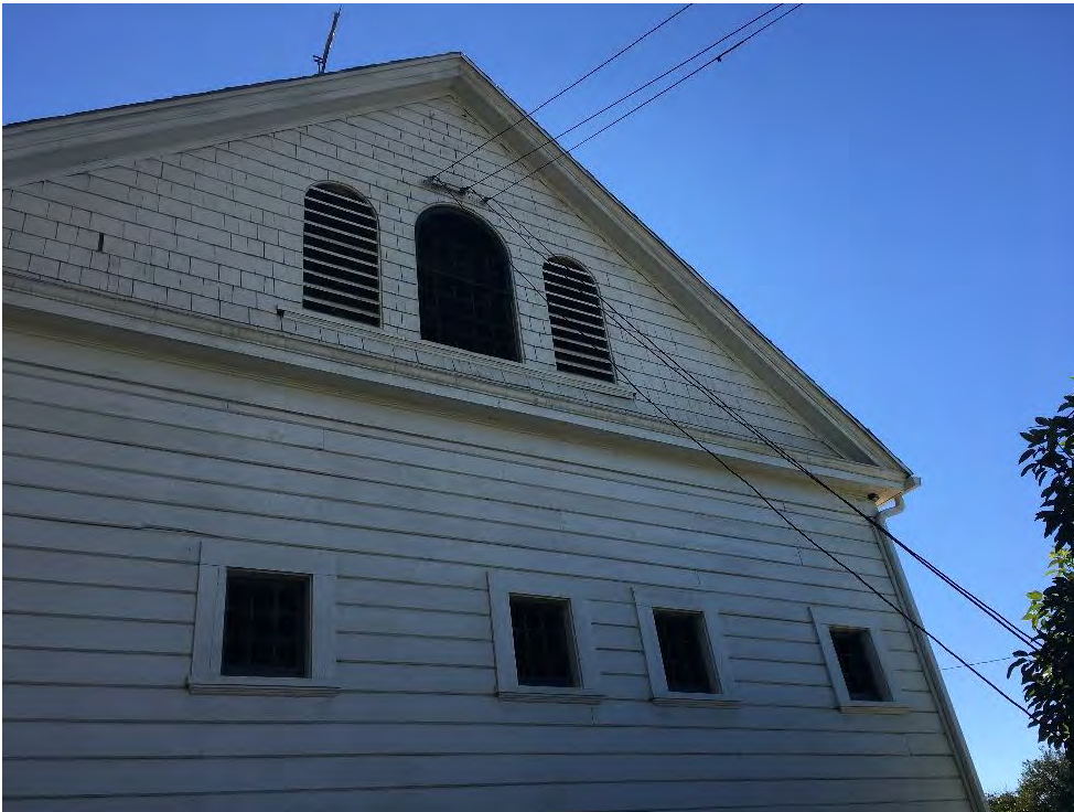
Photograph 8: Northwest elevation of the carriage house with wooden siding and windows visible, flaking white paint, camera facing south, January 9, 2009.
