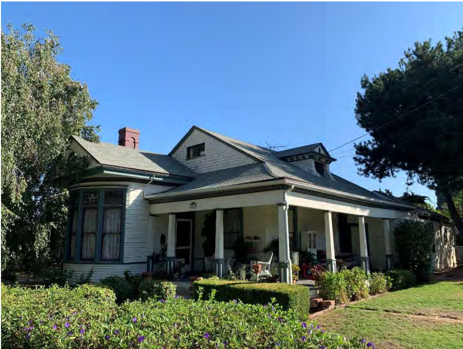
Photograph 2: Overview of southwest and southeast elevations, also in view: front-facing bay window, wraparound porch, decorative window, and sloping roof, camera facing northeast, August 22, 2019.
