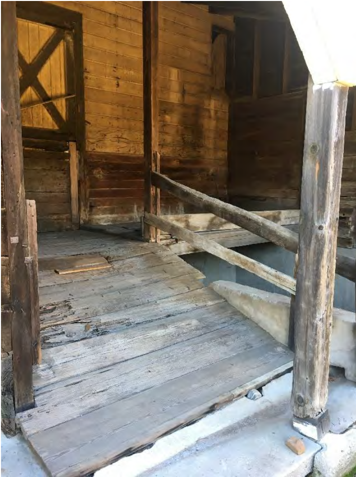
Photograph 5: Detail, wooden walkway leading to back door of carriage house under the covered patio; cement basin also visible on the right side of the photo, January 9, 2019.
