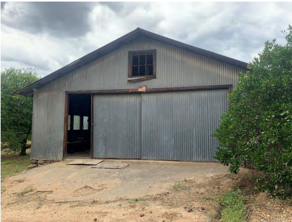
Photograph 5: Southwest elevation, wooden-framed sliding door and windows easily visible, camera facing northeast, July 25, 2019.
