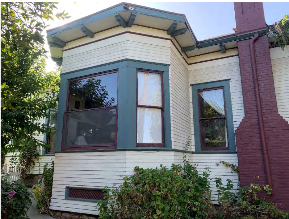
Photograph 5: Detail, second bay window adjacent to channeled brickwork chimney along northwest elevation, August 22, 2019.
