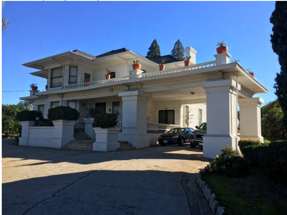
Photograph 2: View of the northwest elevation of the residence and carport from the west side of the semi-circular front driveway, camera facing east, January 9, 2019.
