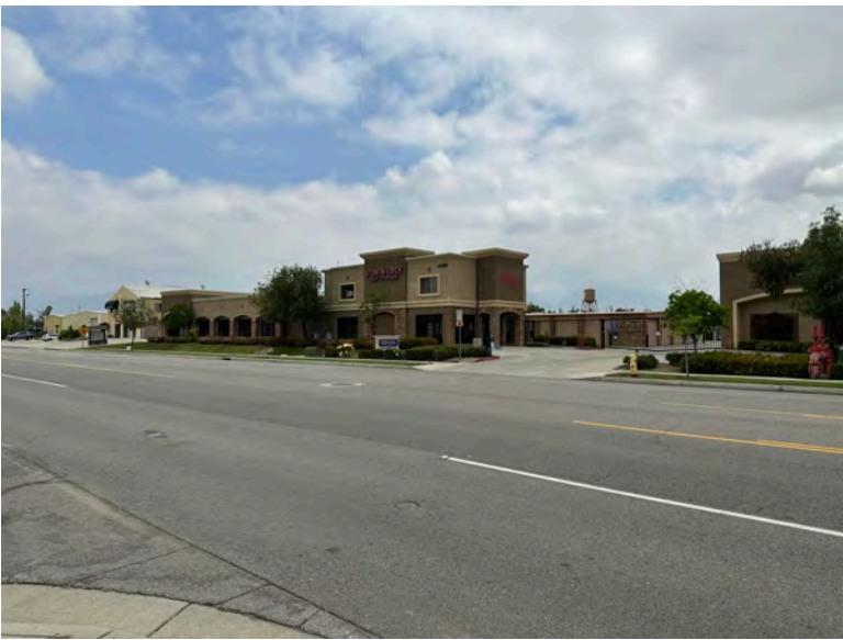
Storage Facility NE of Site
